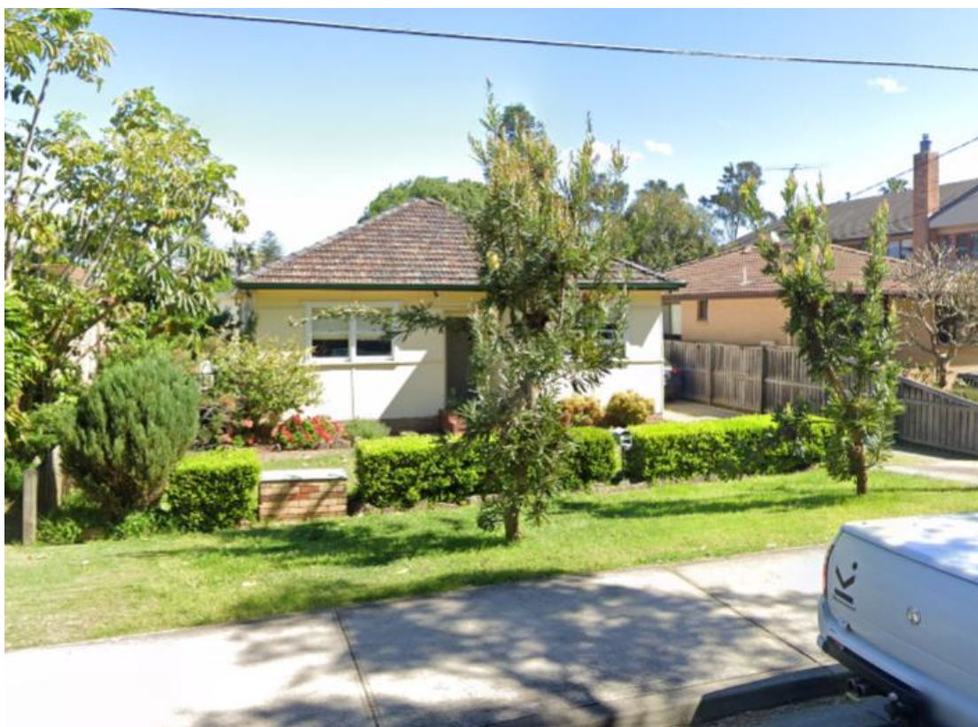
Figure 2 – No. 23 Bassett Street
