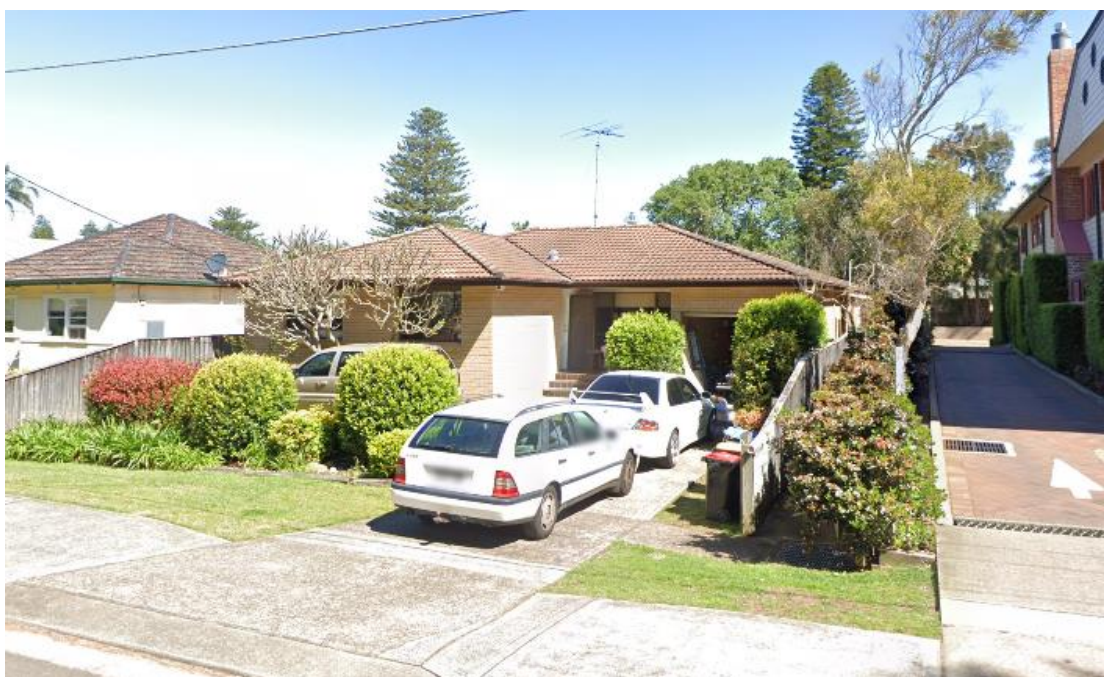
Figure 3 – No. 25 Bassett Street
