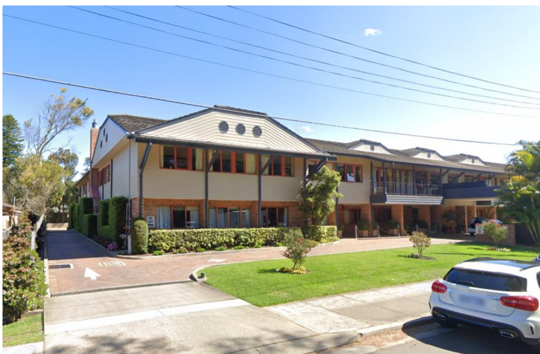
Figure 4 – No. 33 Bassett Street
