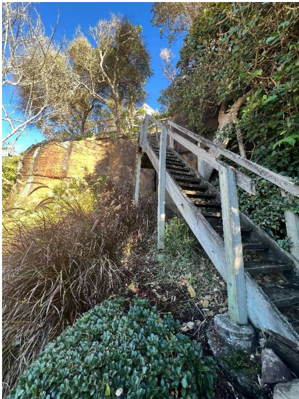
Figure 4 – The existing access stairs (to be relocated to facilitate the proposal) Source: NBP
