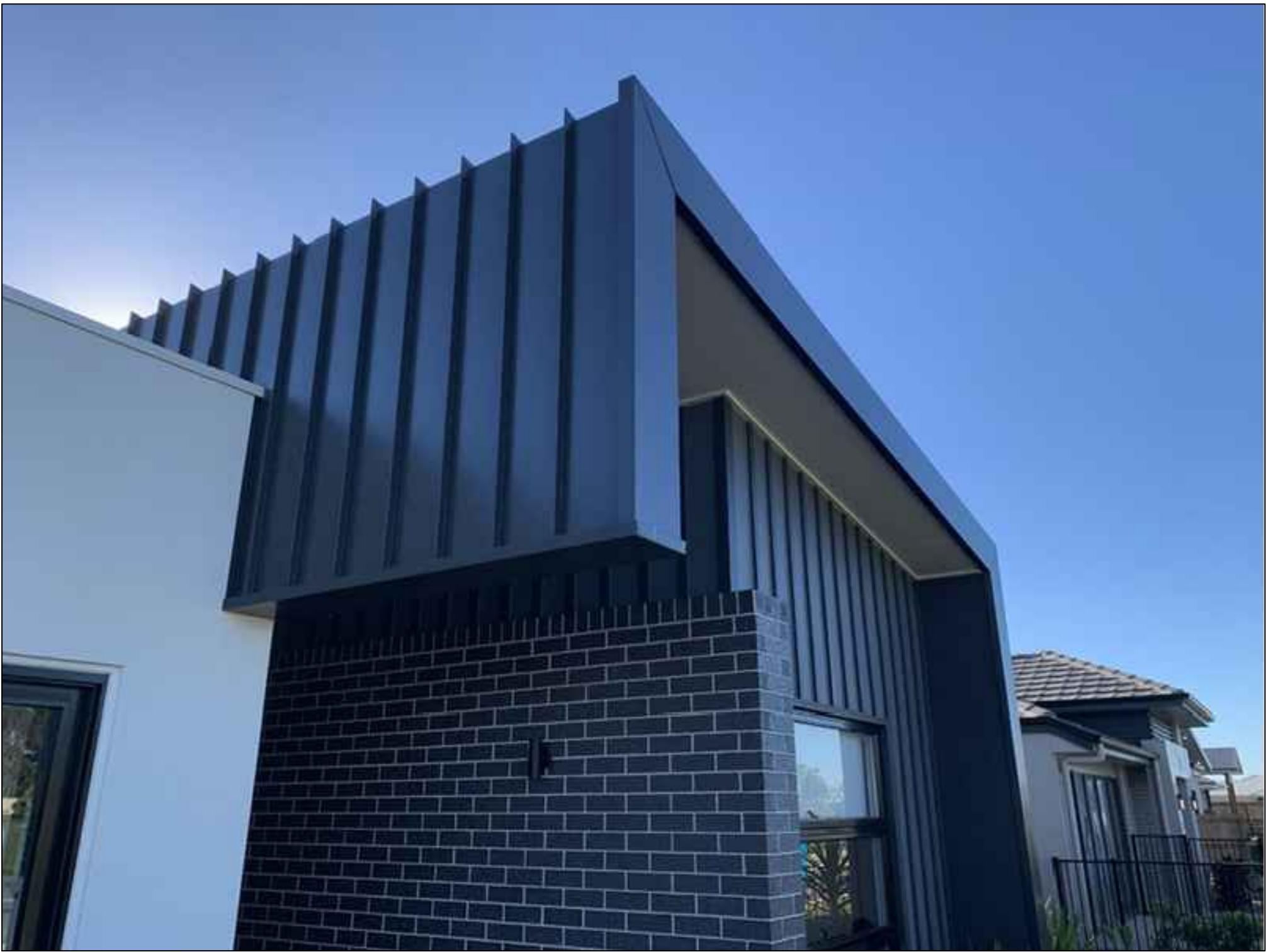
LYSAGHTS LONGLINE COLORBOND SHEETING TO EXTERNAL WALLS COLOUR MONUMENT
