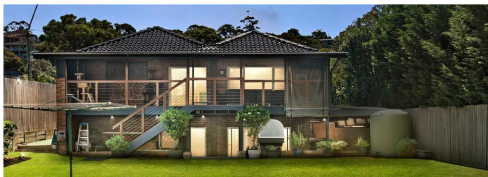
Figure 4 Rear yard view indicating lack of rear retaining wall
