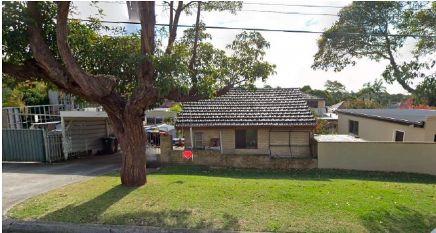
View of Site from the Macmillan Street
