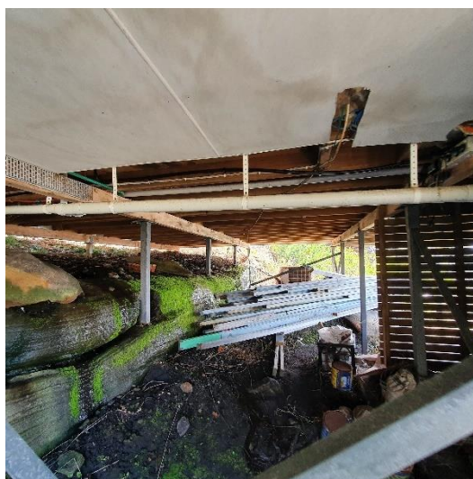
Photograph-4: Secondary dwelling supported by steel columns. View looking north.
