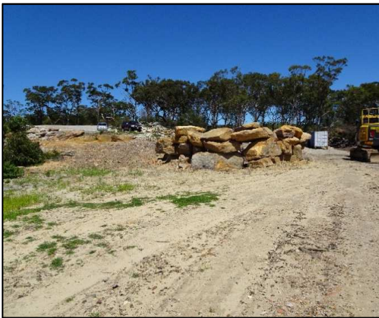
Figure 11. Development site already cleared.
