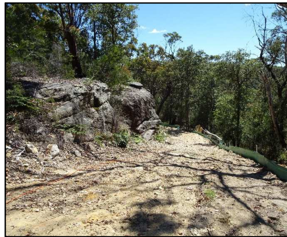
Figure 12. New access road under construction.
