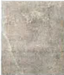
Balcony floor tiles
