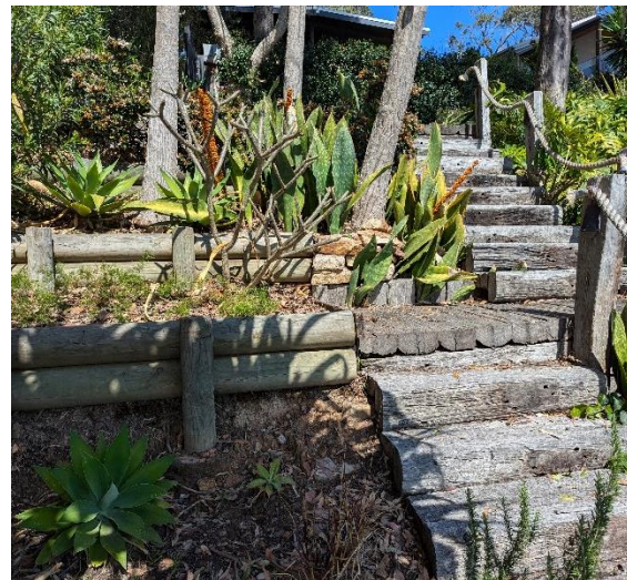
Photograph: 4 – Pathway leading down from existing dwelling to boathouse, including low (<0.40m) timber retaining walls
