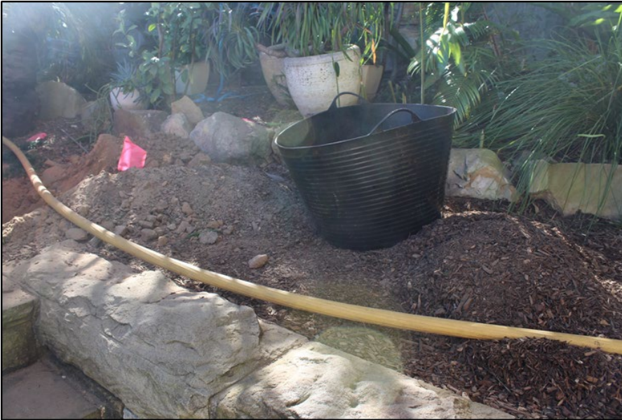
Plate 5 (left) Mulch layer placed to right of plastic bin. Topsoil to left, and subsoil far left. The yellow pipe is the compressed air line for the AirSpade®.
