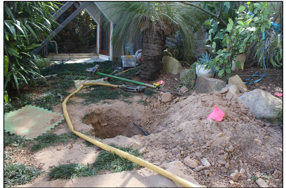
Plate 5 (left) Mulch layer placed to right of plastic bin. Topsoil to left, and subsoil far left. The yellow pipe is the compressed air line for the AirSpade®.
