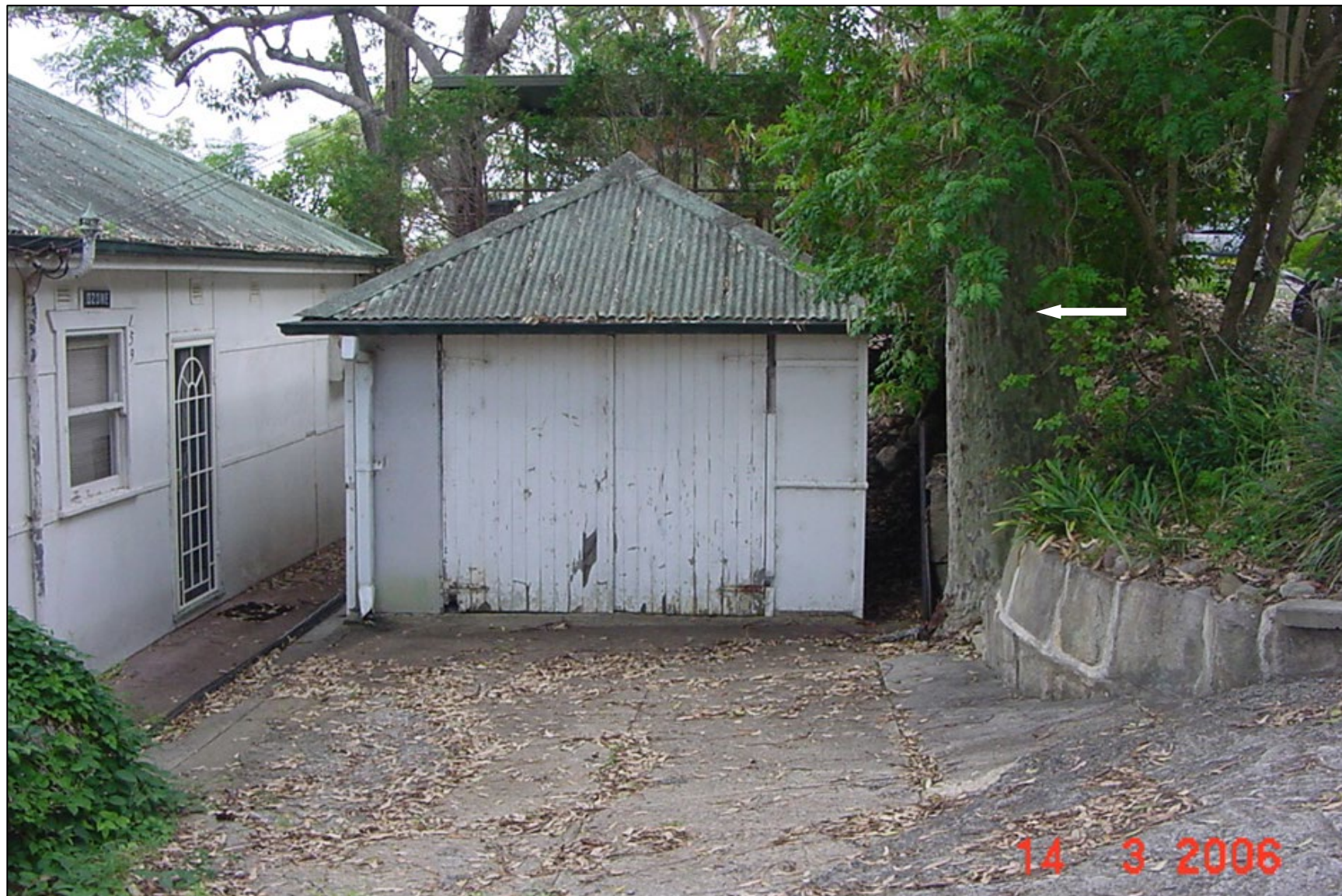
Plate 1 —Illustrates the location of the original dwelling, garage and driveway prior to the more recent construction of the new dwelling. Note the levelled areas supporting the structures. The soil beneath these was consolidated over time. The tree (arrowed) at the base of the original retaining wall. Photo C. Mackenzie. March 2006.
