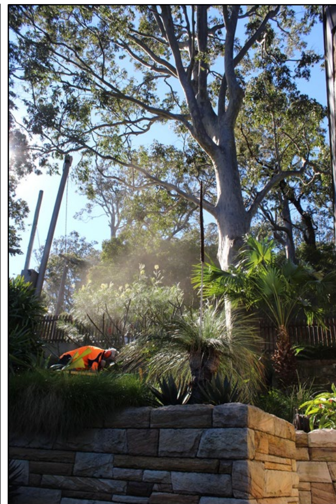
Plate 4 —View of root mapping contractor using the AirSpade® to excavate the pit for the proposed column.
