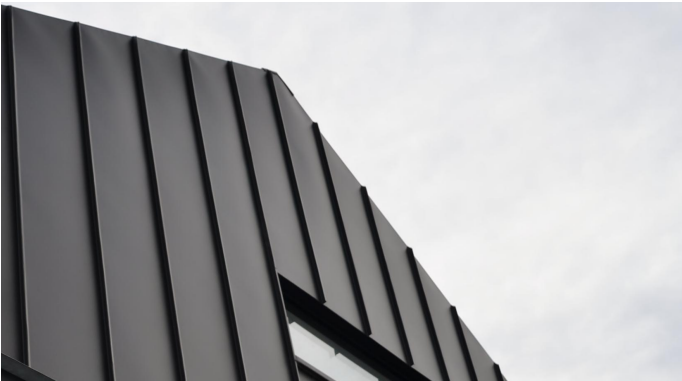
MC1 ALUMINIUM ROOF CLADDING - DARK COLOUR
