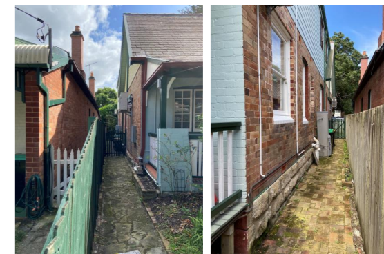
NORTH ELEVATION LOOKING EAST
