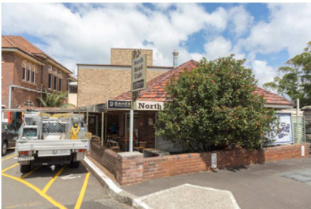
Figure 96: The Kiosk, Building 5 from the north.
