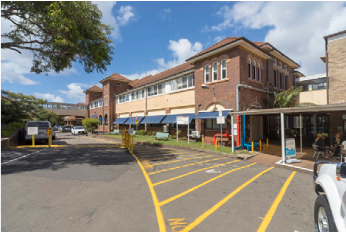
Figure 44: The western end of the north elevation of Building 1 and the west elevation (right) of Building 1, and junction with Building 3
