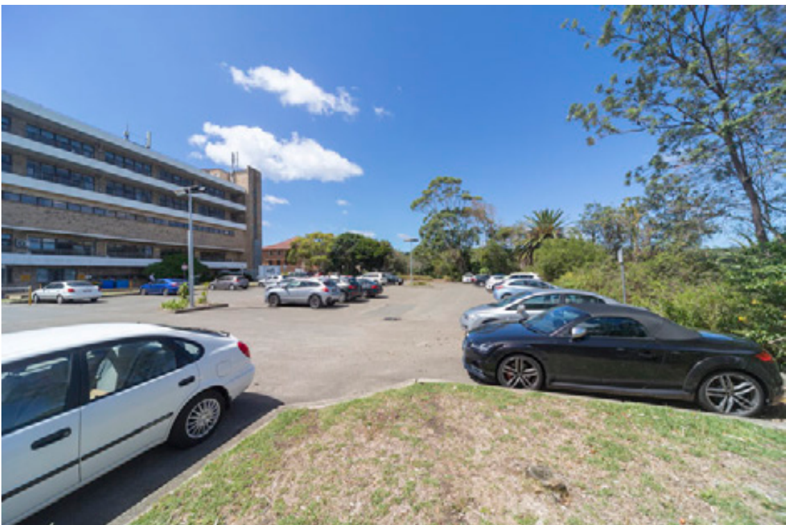
Figure 117: View across the southern end of the site from the west looking east, with Building 4 to left and car parking area P1
