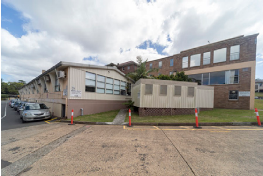
Figure 106: Building 21 at left, Building 22a at right, with Building 22 just visible beyond (centre, background)
