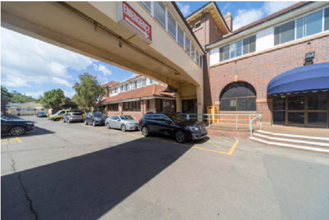
Figure 42: Eastern end of the north elevation of Building 2, taken from the west looking east, with bridge link to Building 1
