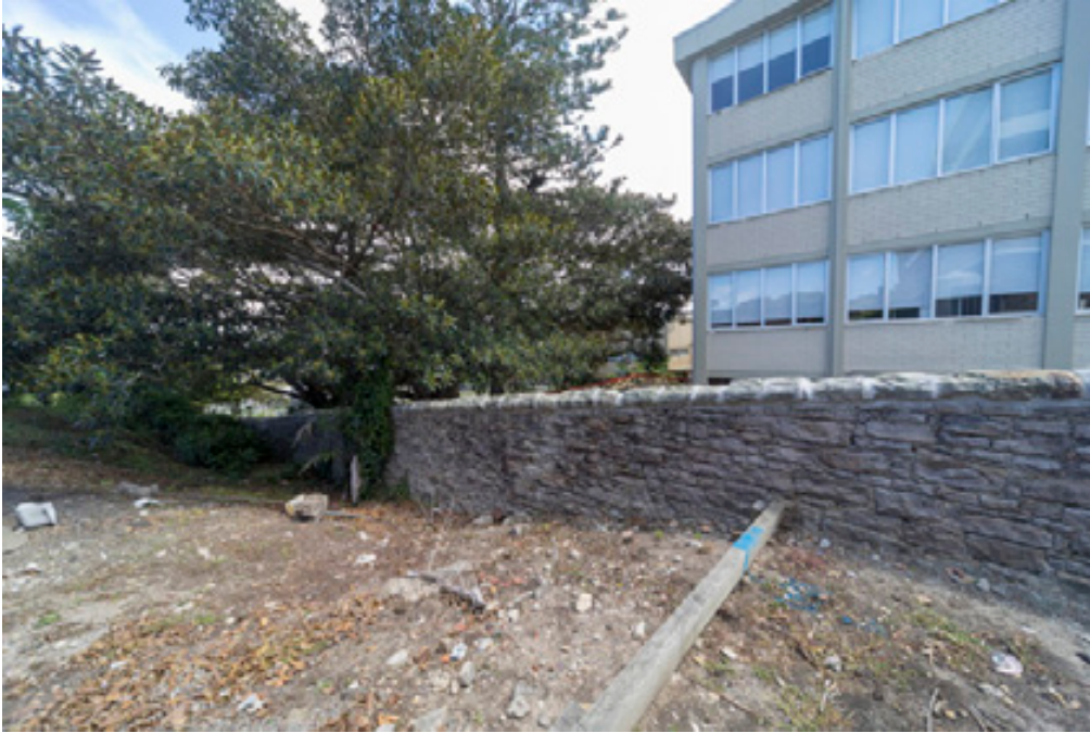
Figure 39: Detail of western boundary wall of the core hospital site, showing use of the hard white cement mortar, particularly to the capping stones.
