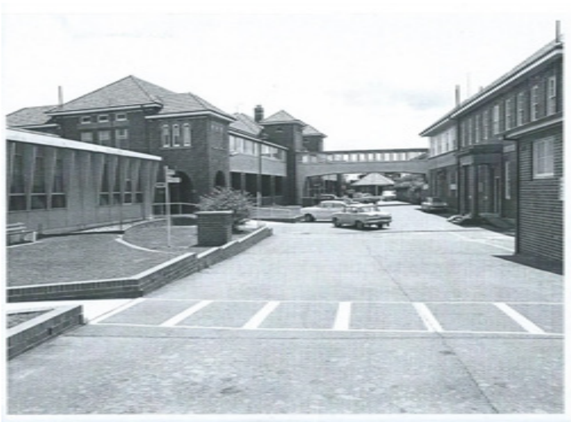
Figure 20: Main Ward Block (Building 2) and Maternity Ward (building 11) in 1969, (at left) with the rear of the 1928 Administration & outpatient's building 1 at right (prior to later alteration). This also shows the bridge built prior to 1959 between Buildings 1 and 2. Source: Local Studies Collection, Manly Library.
