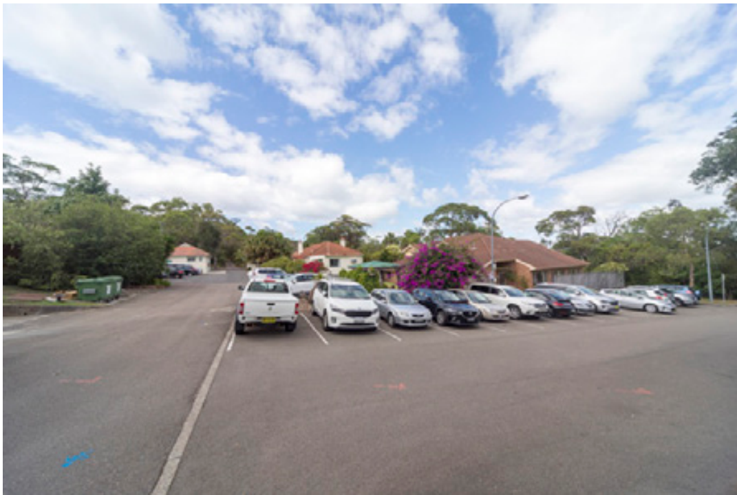
Figure 105: Looking east from car parking area P5, with the stables and Building 20 at left, with Building 35 (constructed 1996) at right. Building 35 is the most recent building constructed at Manly Hospital.
