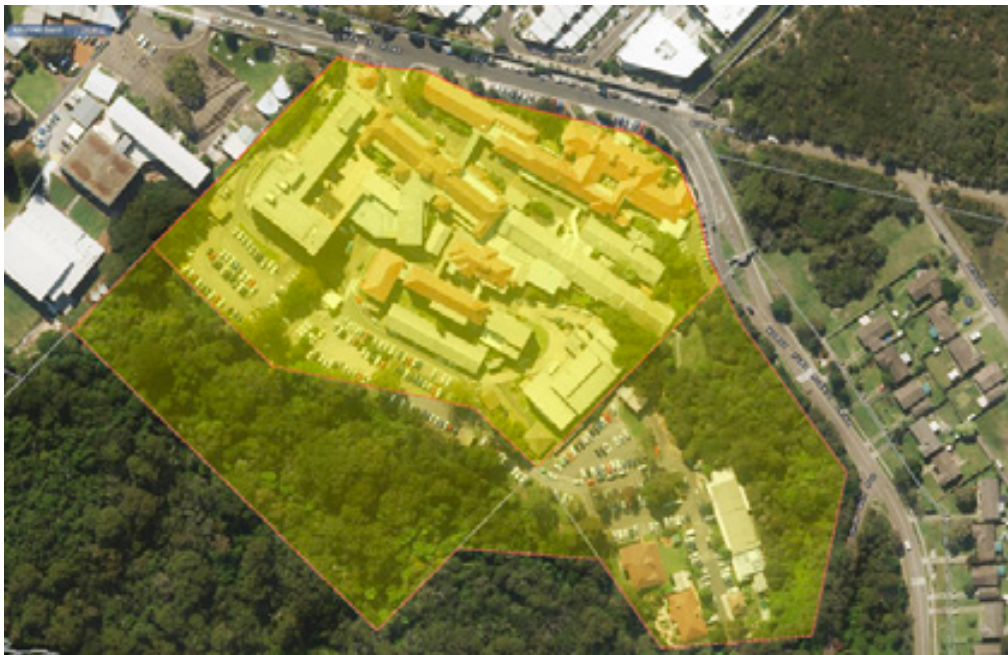
Figure 2: Recent satellite view of all four lots of the Manly Hospital site (shaded yellow, outlined in red Source: NSW Land & Property Information (LPI) Six Maps
