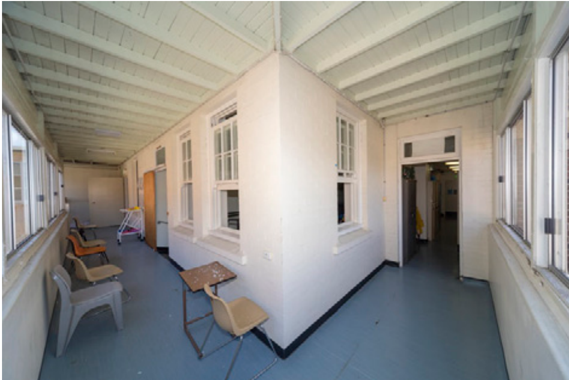
Figure 58: South-east corner of Building 15 with original windows and timber verandah ceilings
