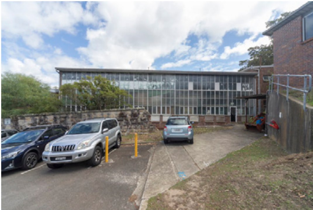
Figure 33: Another view of the eastern boundary wall from the east with Building 13 beyond.
