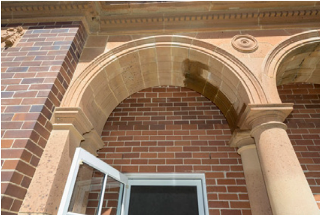
Figure 102: Detail of sandstone arches to the remnant façade of Building 1. Note the wall visible beyond is part of 1992 alterations and additions which included construction of Building 30 to the east.
