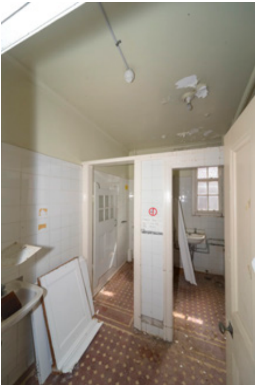
Figure 68: (Left) Original bathrooms to Level 1 Building 22 including tessellated tiling
