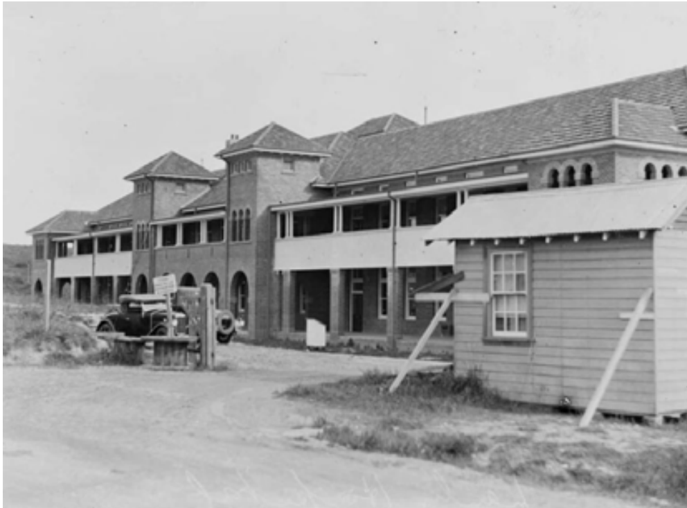
Figure 13: 1928 photo of the rear of the Main ward block (Building 2). Source: Fairfax photo sourced from NLA Trove
