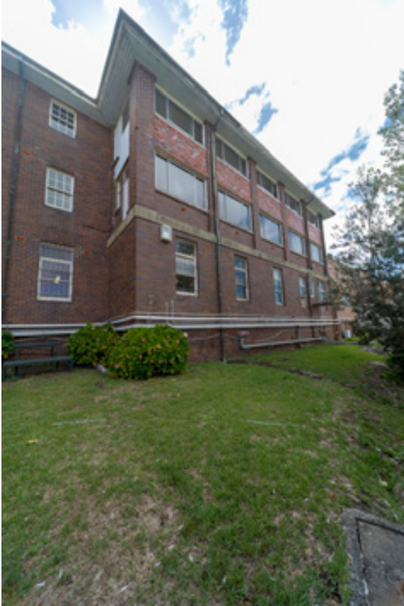
Figure 59: (Left) south elevation of Building 22 Kalori (former nurses' home)
