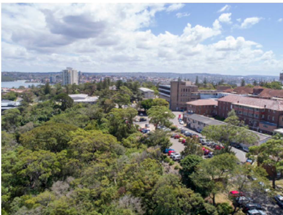
Figure 31: Drone photo of the western end of the Manly Hospital building complex from the south, with Building 22 (3 storeys) and Building 21 (1 storey) at far right, and the 5-storey Building 4 (arrowed) just right of centre.
