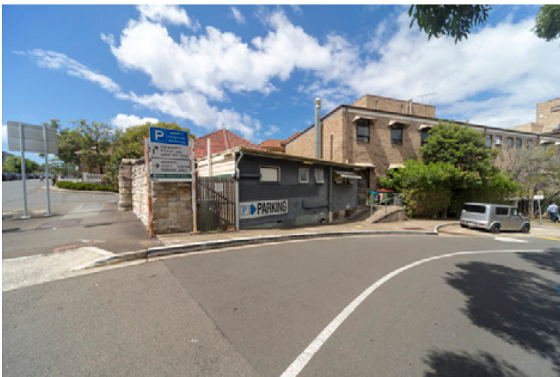
Figure 99: The Kiosk from the west (roof arrowed), with later additions, and Building 3 at right. Note the sandstone wall to the north of the Kiosk appears to be of recent construction.
