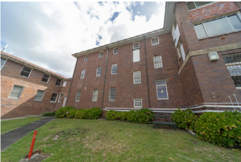
Figure 60: Western end of the south elevation of Building 22 Kalori, showing at left Building 22A and junction with Building 22A
