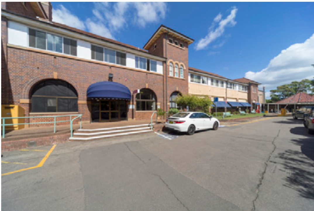
Figure 40: The western end of the north elevation of Building 2 with Kiosk (Building 5) at far right. Note roughcast stuccoed balustrading remains to balconies at right, however all balconies have been enclosed, and the arched colonnade infilled with aluminium framed windows.
