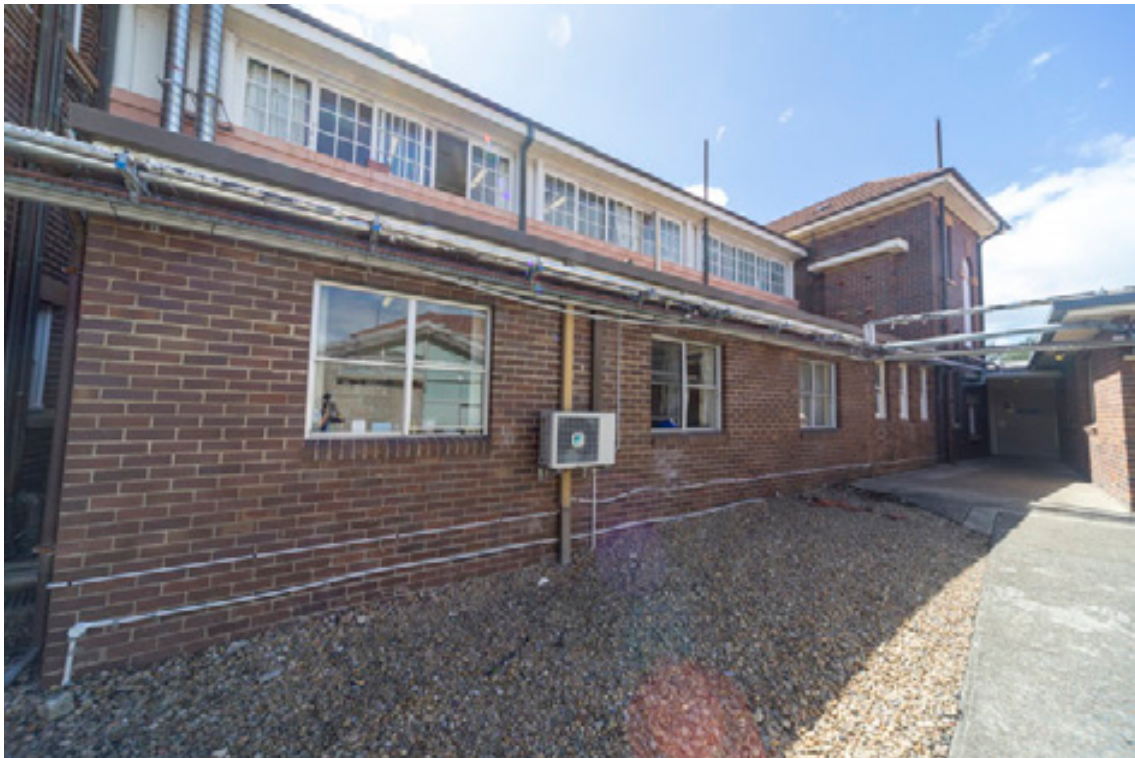
Figure 45; Part of the south elevation of Building 2
