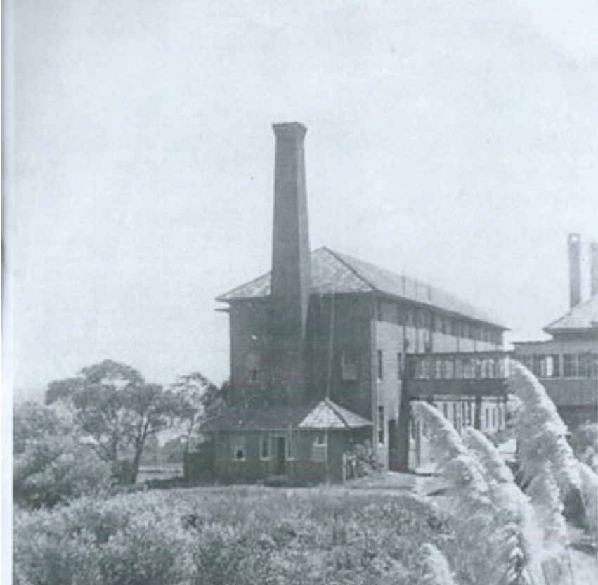
Figure 17: A 1949 photo of the eastern end of the 1931 Nurse's home showing the Boiler House and chimney and the northern elevation. Source: Local Studies Collection, Manly Library
