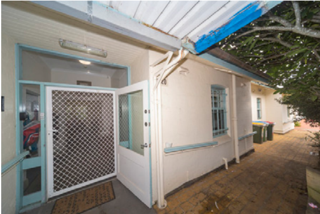
Figure 76: The entry area and western end of the north elevation of Parkhill cottage. Note modern door, fanlights and sidelights to entry area.
