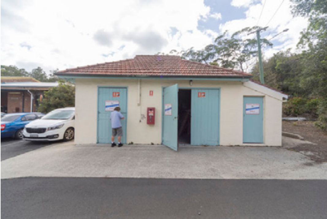
Figure 90: South elevation of the stables to Parkhill cottage (Building 20). The skillion section to the right (east) is clearly a later addition to the stables.
