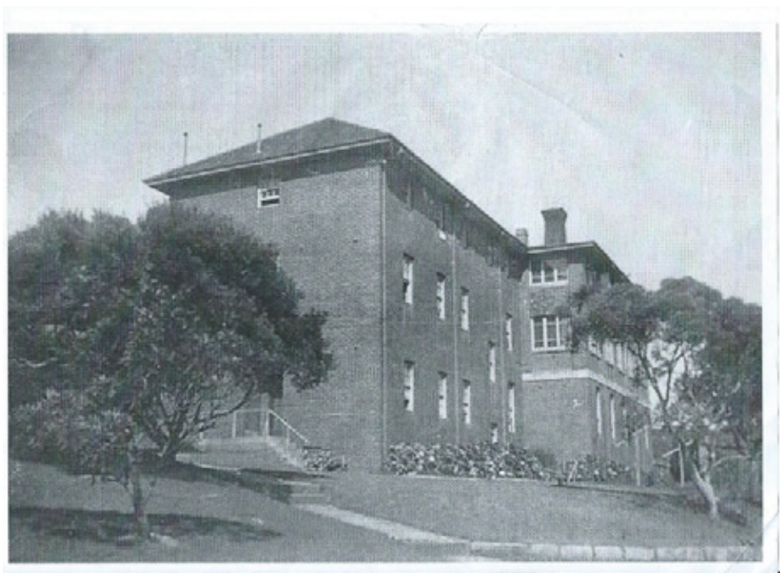
Figure 16: A 1949 photo of the 1931 Nurses' Home, photo taken from the south-west, showing western and southern elevations. Source: Local Studies Collection, Manly Library
