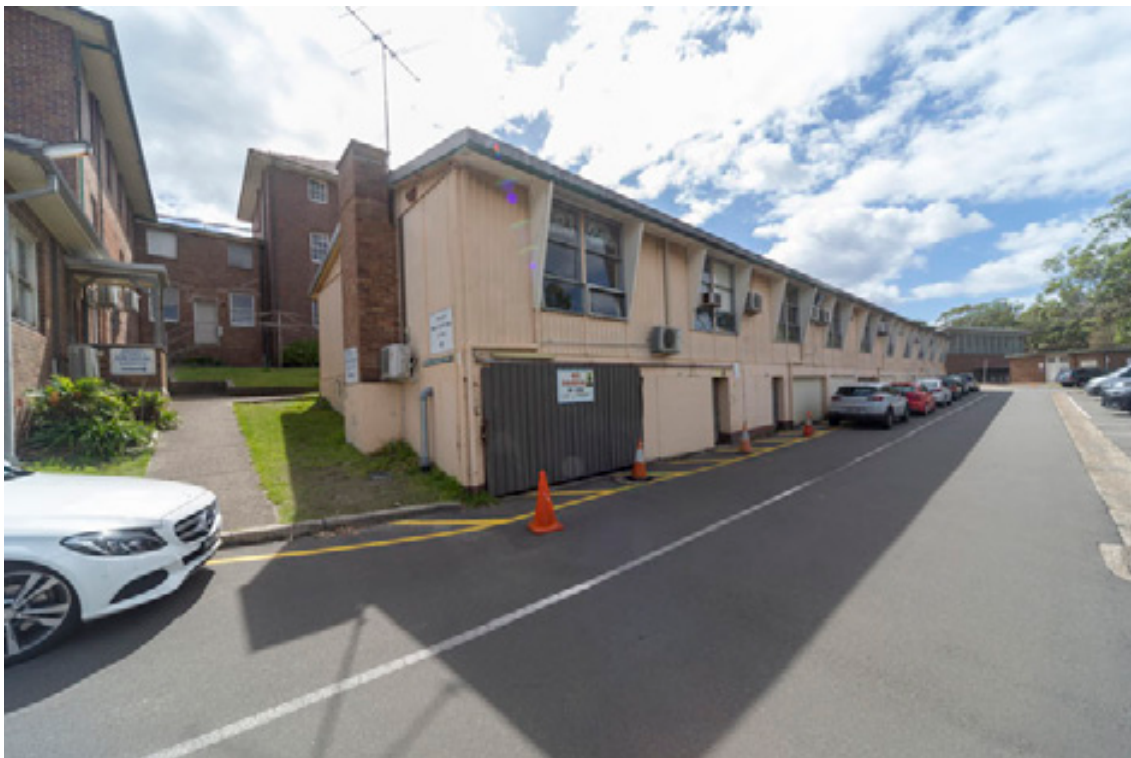
Figure 107: View of the western end of Building 21 with Building 22A at left, and Building 22 just visible beyond Building 21 (centre, background, arrowed)
