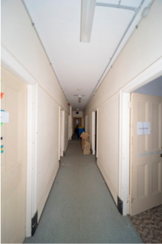
Figure 67: (Left) corridor, Building 22 Level 1 interior including original doors, joinery
