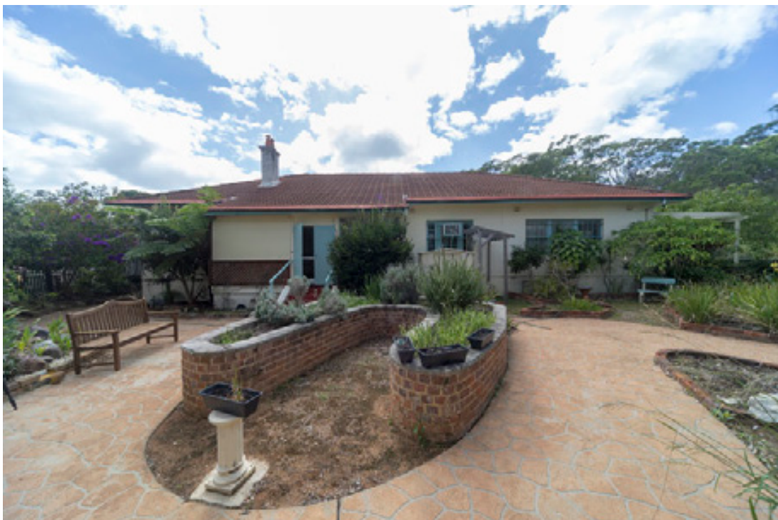
Figure 81: The south elevation of Parkhill cottage. Note concrete roof tiling however the chimney remains.
