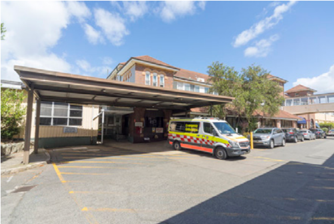
Figure 43: Eastern end of the north elevation of Building 2, looking west, with Building 11 at far left, bridge link to Building 1 at far right
