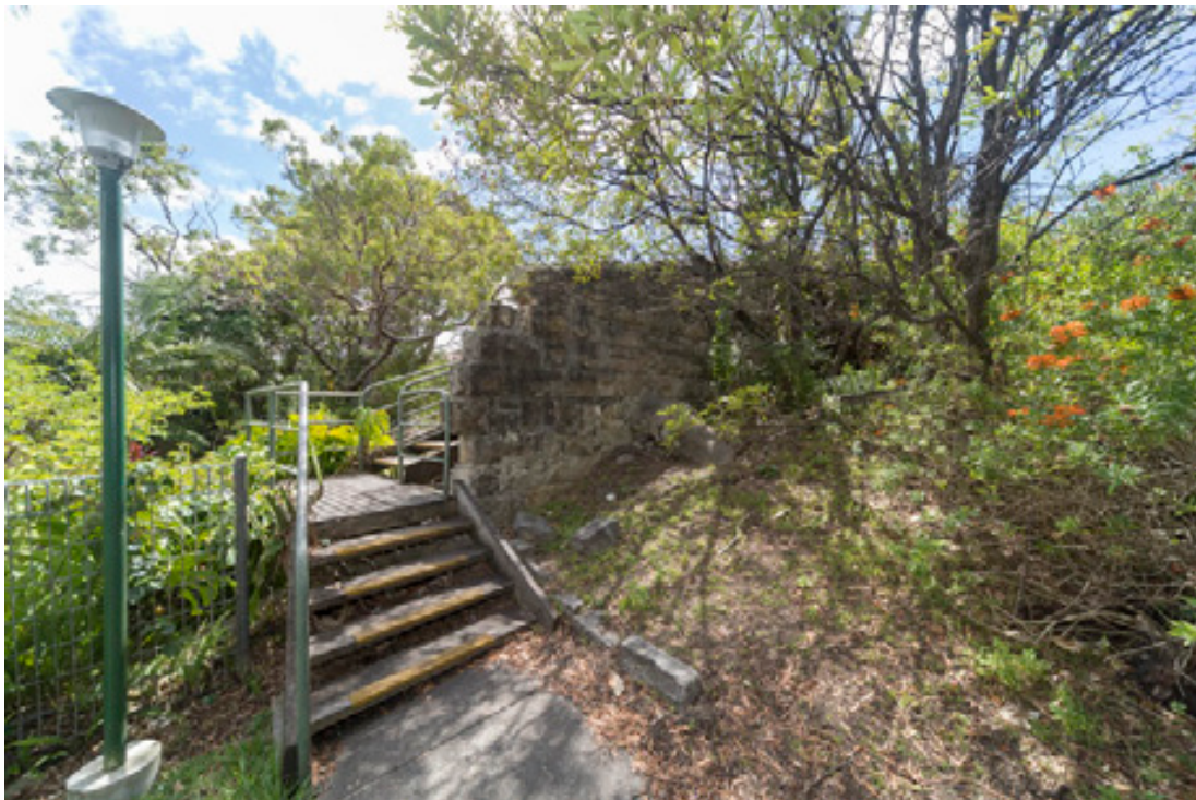
Figure 36: Steps from Car parking area P6 and view of the eastern side of the northern end of the eastern boundary wall of the core hospital site.
