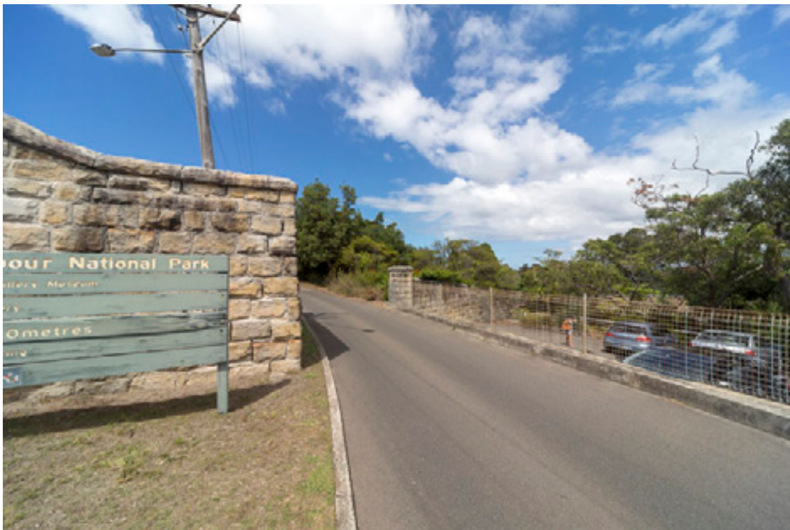
Figure 34: View of the northern end of the eastern boundary wall, adjacent to Car parking area P6 (arrowed)
