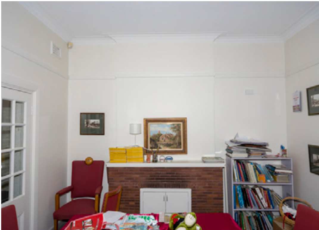
Figure 84: Picture rail, cornices and chimney breast to Parkhill cottage interior
