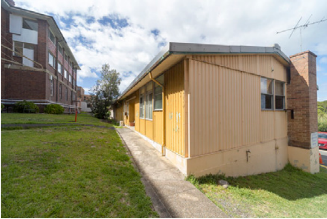
Figure 108: View of the area between Building 22 (left) and Building 21 (right).
