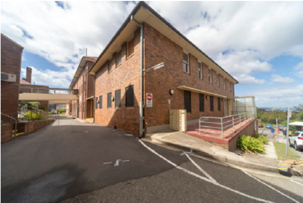
Figure 62: View from looking east between Building 22A, with Building 22 beyond, and bridge link into Building 15 at left
