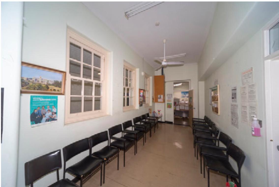
Figure 55: Waiting area on northern side of Building 15 with original windows to the northern wall.
