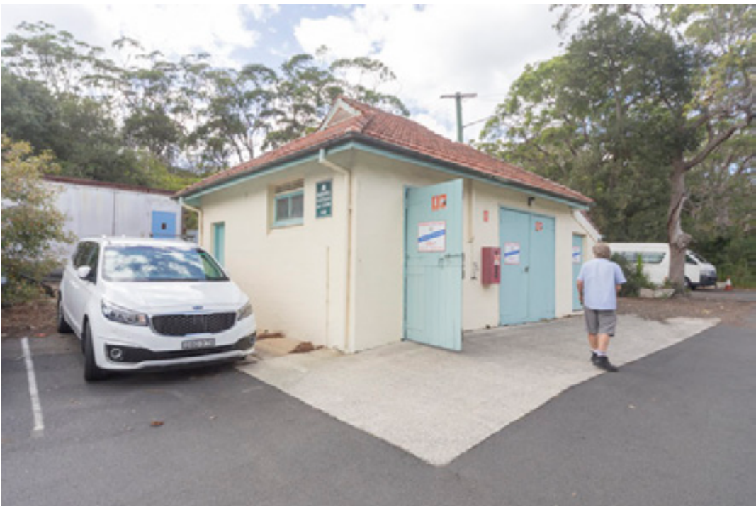
Figure 91: The stables to Parkhill cottage (Building 20), west and south elevations, showing original timber ledged and braced doors and original terracotta tiled roofing.
