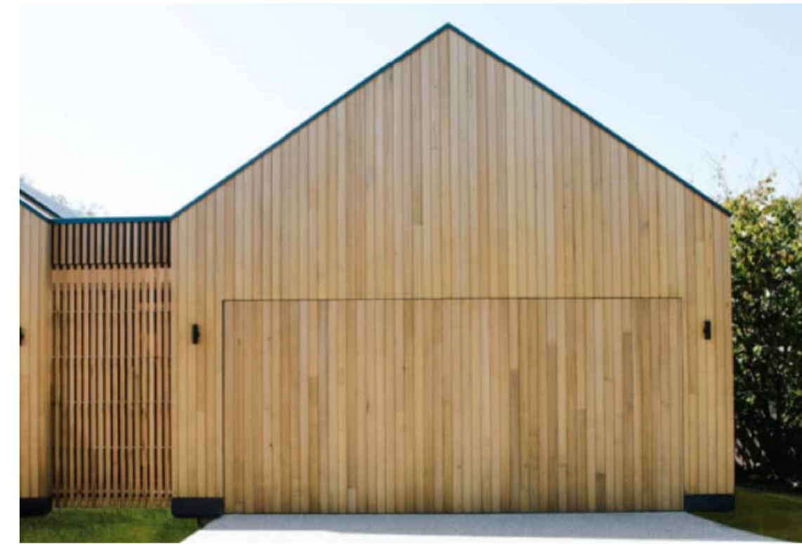
VERTICAL TIMBER CLADDING
