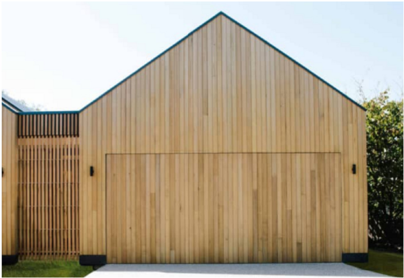
VERTICAL TIMBER CLADDING
