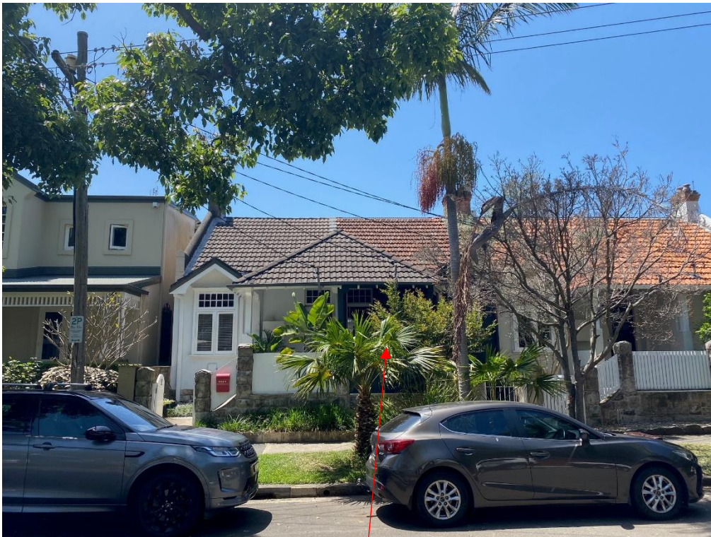
Photograph of the subject site – 10 Smith Street, Manly
