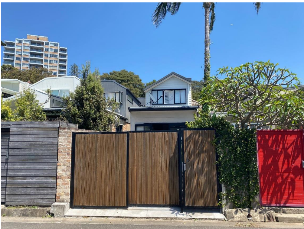
Photograph of the site from the rear lane
