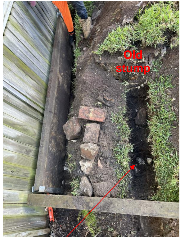
Image o: Trench 2- loose rubble and large amount of dead and decomposing roots from the large stump beside
