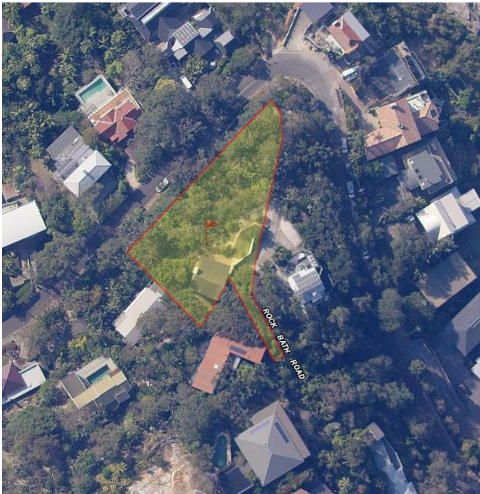
Figure 1: Site Location (Source: Six Maps)
