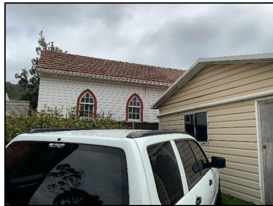
Figure 26. Detail of St Michaels Anglican Church as viewed from the rear of the subject site.
