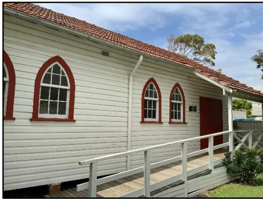
Figure 23. Detail of the façade of St Michaels Anglican Church.
