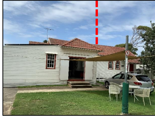
Figure 22. Façade of St Michaels Anglican Church. The subject site, behind, is approximately located to the right of the dashed line.
