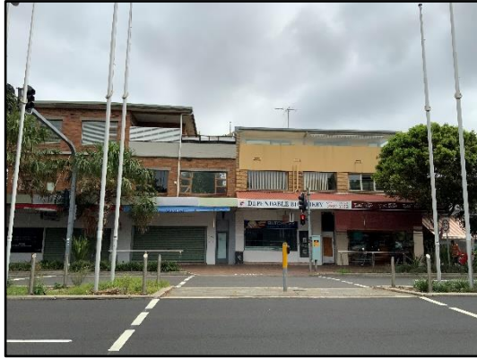
Figure 15. Primary façade of subject site as viewed from Barrenjoey Road.
