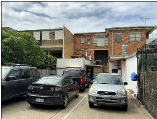
Figure 17. Rear elevation of subject site as viewed from external hardstand area.
