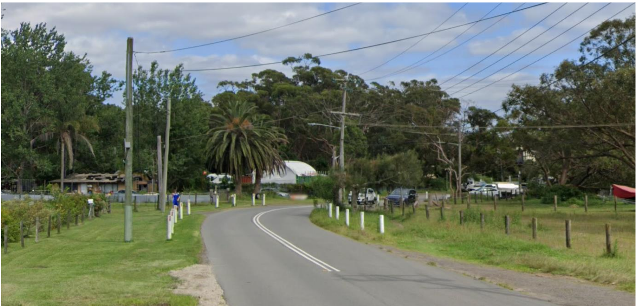
Figure 2: Boondah Road (looking north)
