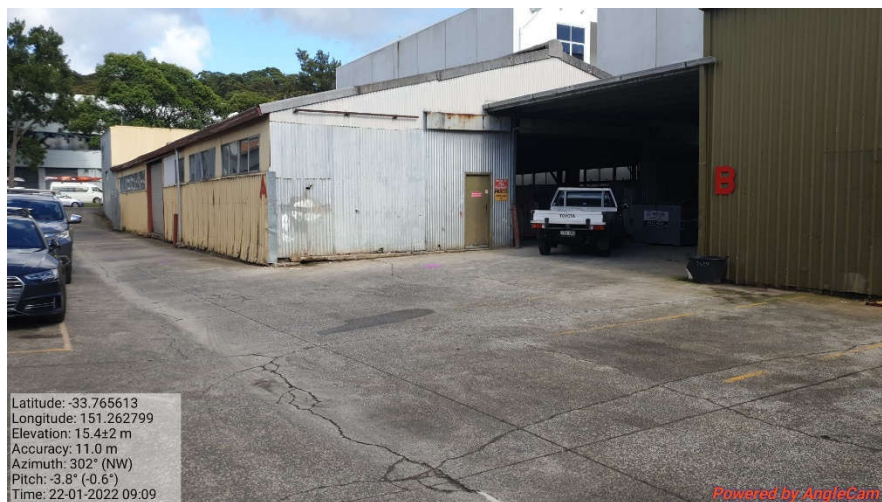
Photograph 3: Cracked pavement and drain
