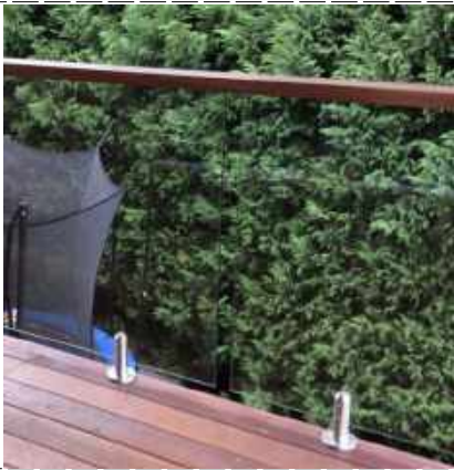
Glass balustrade with timber handrail
