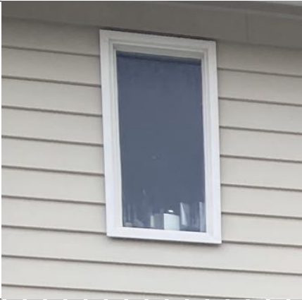
Painted timber window to kitchen
