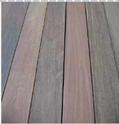
Timber treads to external stair
