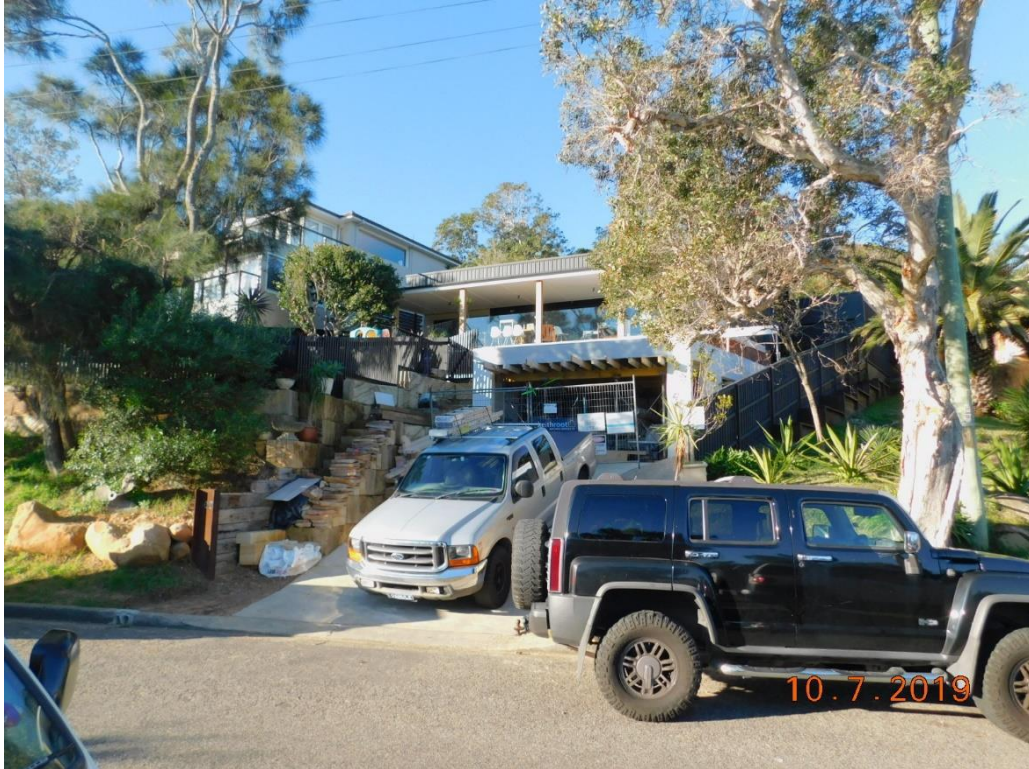
Fig 3: View of subject site, looking north-east from Marine Parade
