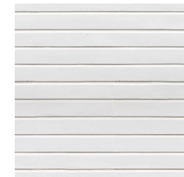
LIGHT COLOURED CLADDING
