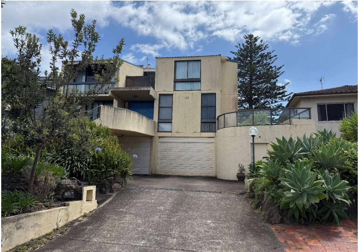
Figure 7 – A three storey dwelling at 16 Hillcrest Avenue Source: NBP
