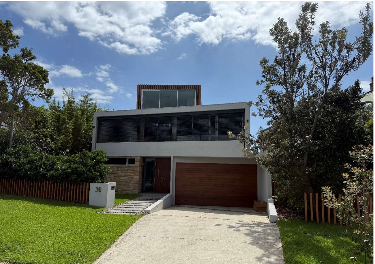
Figure 6 – A three storey dwelling at 30 Hillcrest Avenue Source: NBP
