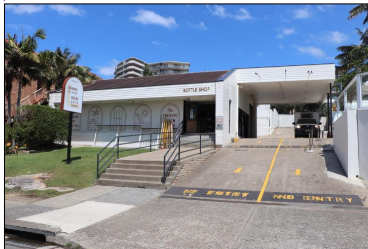
Figure 31: The front (northern) elevation of No. 31 Moore Road, Freshwater.
