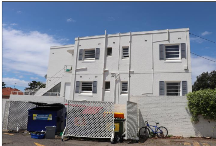
Figure 34: The western elevation of No.64 Undercliff Street, Freshwater
