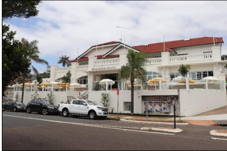
Figure 20: The front (northern) elevation of No. 29 Moore Road, Freshwater.
