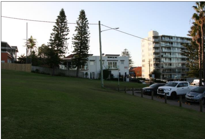
Figure 47: The Harbord beach Hotel is not visible from No. 80 Undercliff Road, Freshwater
