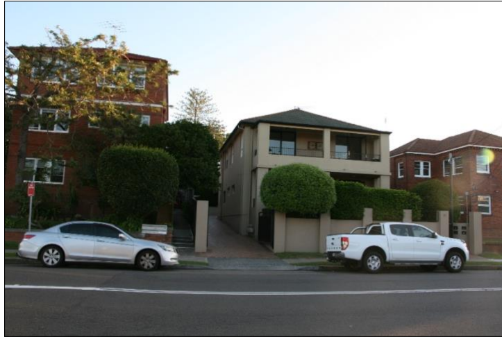
Figure 37: Typical built form of Moore Road.
