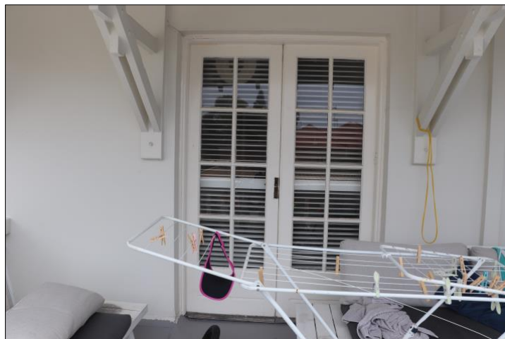
Figure 27 Timber framed doors to the eastern elevation.
