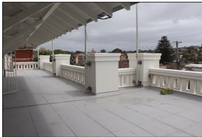
Figure 24: The rear of the masonry balustrade.
