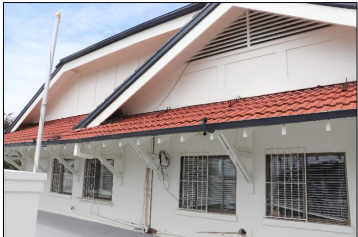
Figure 22: Detail of tiled verandah roof and sliding aluminium framed windows.
