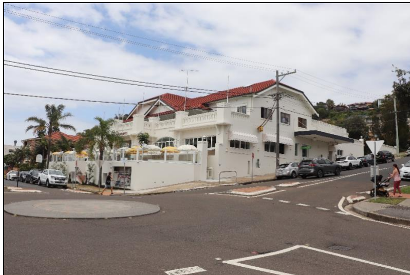
Figure 42 View of the building from the west.
