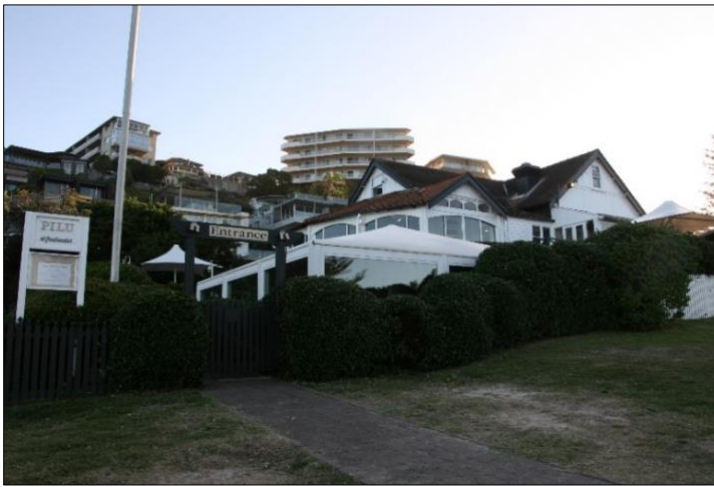
Figure 46: No. 80 Undercliff Road, Freshwater.
