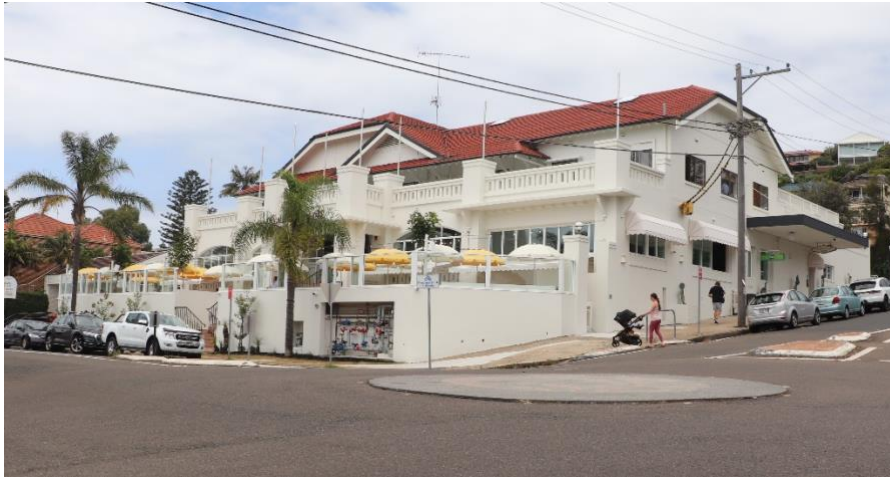
Figure 17: Current external appearance of the building January 2021.
