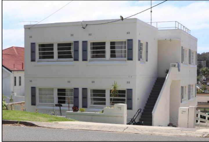
Figure 33: The front (southern) elevation of No. 64 Undercliff Street, Freshwater.
