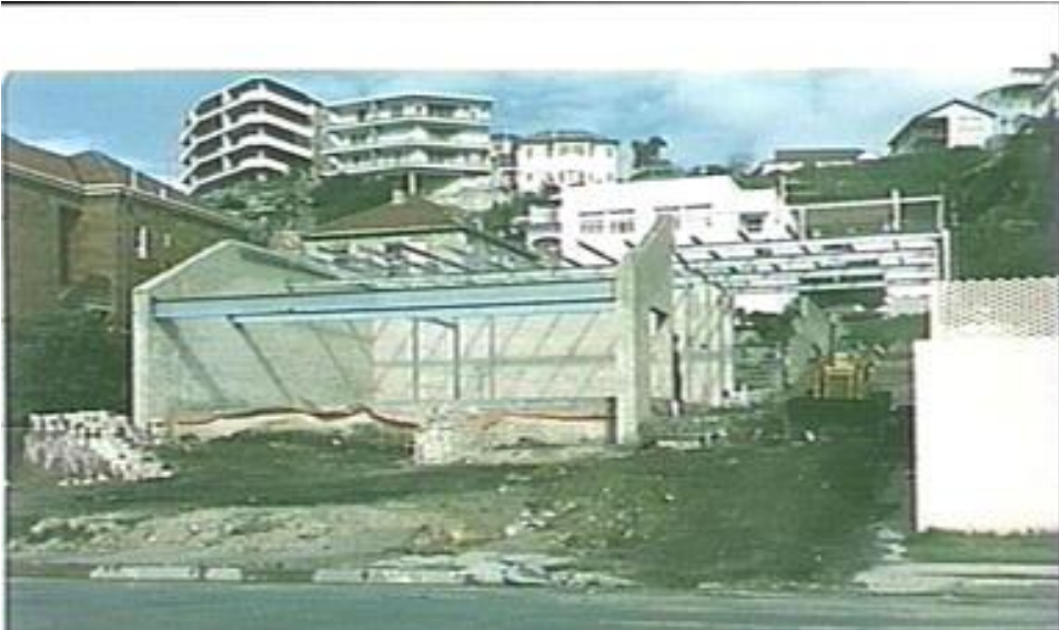
Figure 16: Construction of the bottle shop, 1982 Northern Beaches Local Studies ref: 40\WAR40544
