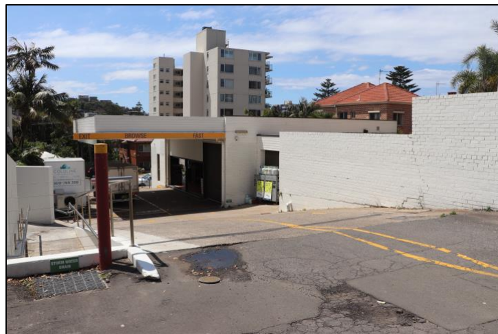
Figure 32: View to the rear of the building form within the site.
