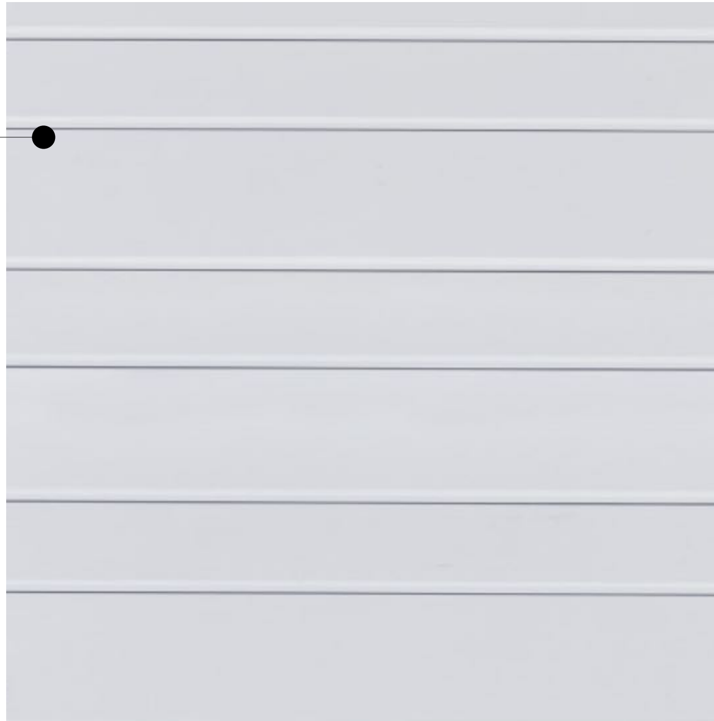
NEW PUBLIC TOILETS WALL - FERRY TERMINAL SIDE WHITE PAINTED HORIZONTAL PROFILED CHAMFER BOARD CLADDING IN 2 WIDTHS TO MATCH EXISTING EXTERNAL CLADDING
