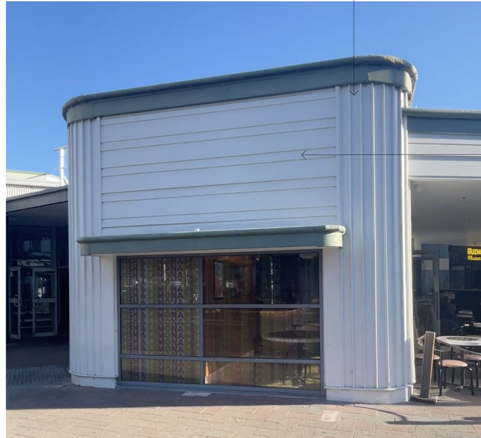
NEW PUBLIC TOILETS WALL - FERRY TERMINAL SIDE WHITE PAINTED CFC SHEET WITH VERTICAL PAINTED TIMBER BEADS TO 400mm RADIUS CORNER
