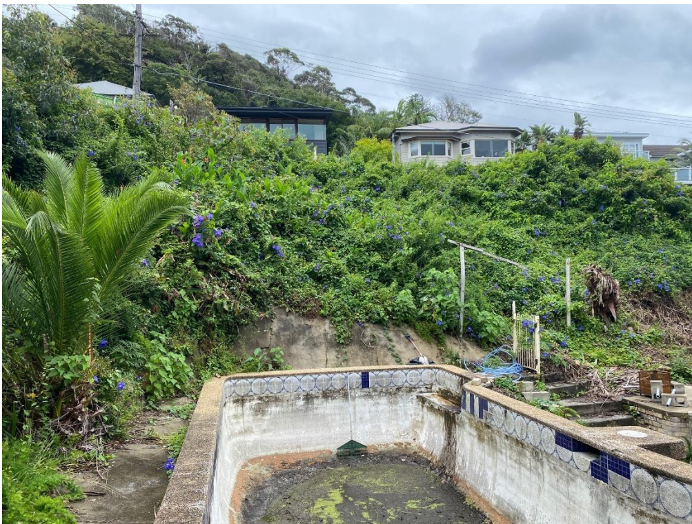
Photograph of existing pool area and structures looking west – note no visual impacts to the street
