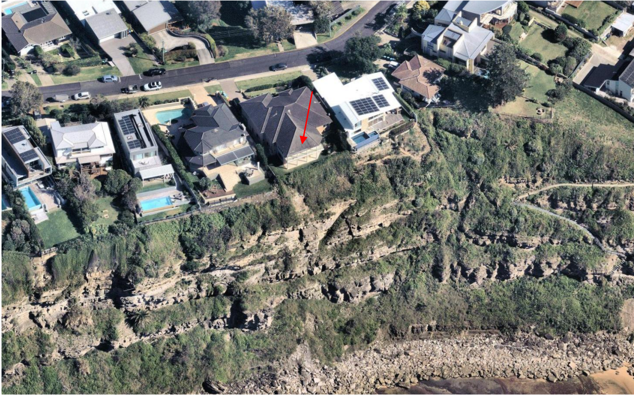
Figure 2: Oblique aerial view of site (at arrow) on 1 May 2023, facing west
