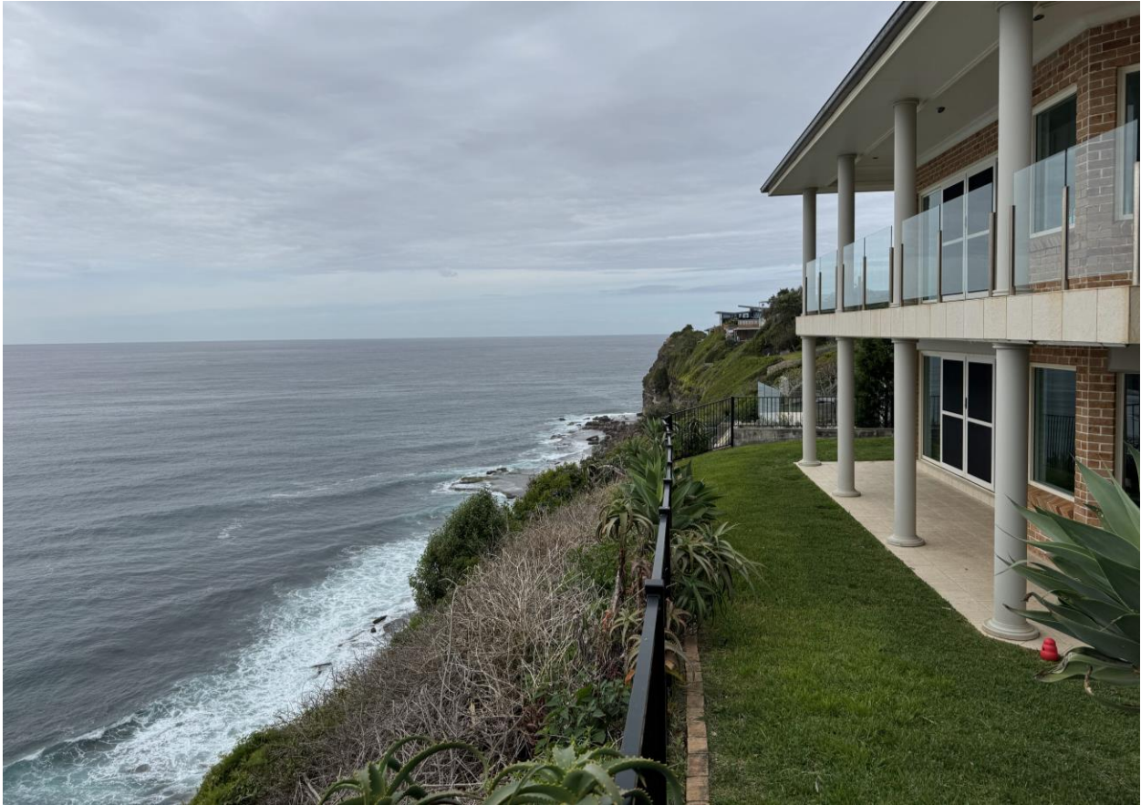
Figure 4: View of seaward face of dwelling at site on 16 October 2024, facing SSE
