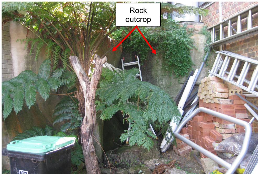
Photograph 10 – View along the eastern side of the residence at 16 Marshall Crescent (towards the north), showing a sandstone outcrop passing through the site. Both residences on 16 Marshall Crescent and 17 Marshall Crescent appear to be founded on the rock outcrop at this location.
