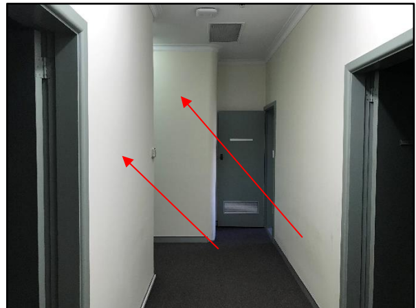
Figure 28. View to the internal corridor. The red arrows indicate the curved masonry walls.
