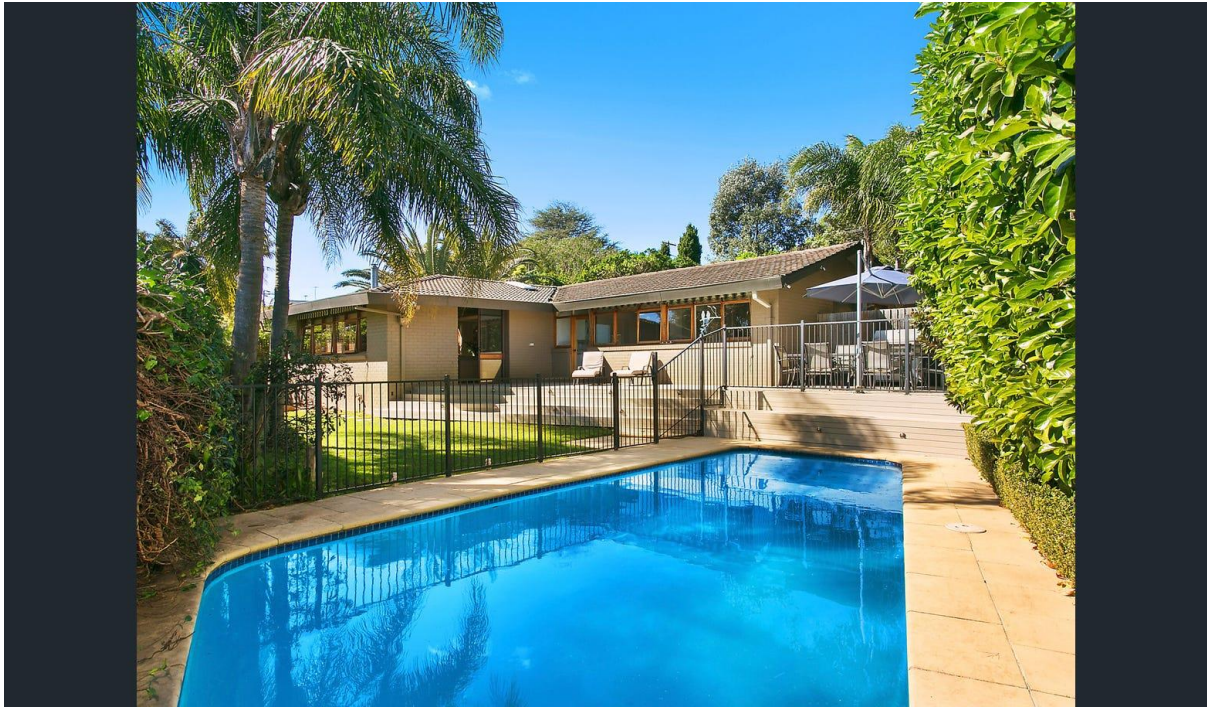
VIEW LOOKING TOWARDS THE REAR OF THE DWELLING – PROPOSED FIRST FLOOR ADDITION
