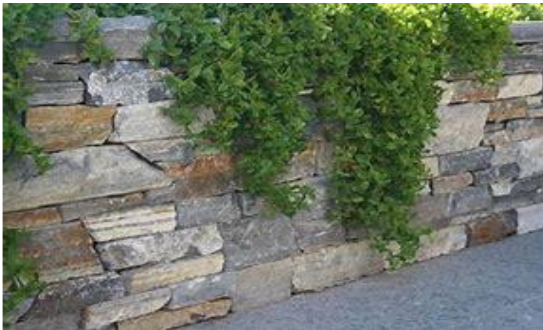
STONE WALL CLADDING
