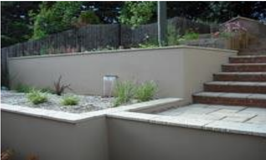
RENDERED MASONRY WALLING
