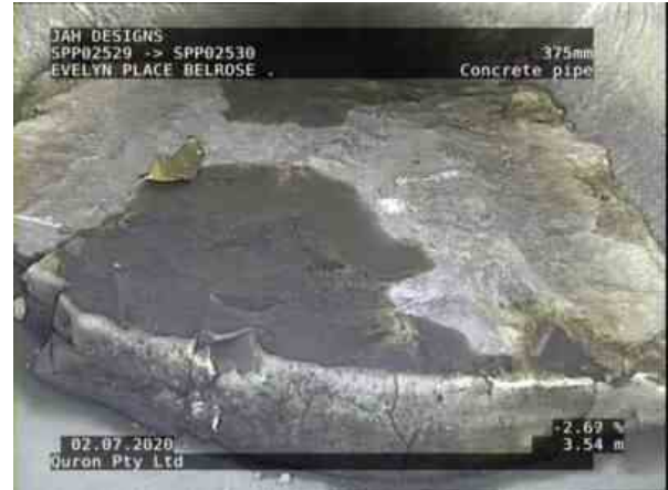
SPI01992_ea245793-be85-4723-9209-d3fc2e3f99bb_20200702_122349_851.jpg, 00:01:46, 3.54 Deposits in the invert, hard compacted material, concrete, Obstruction: 5-20% from 5 o'clock to 7 o'clock
