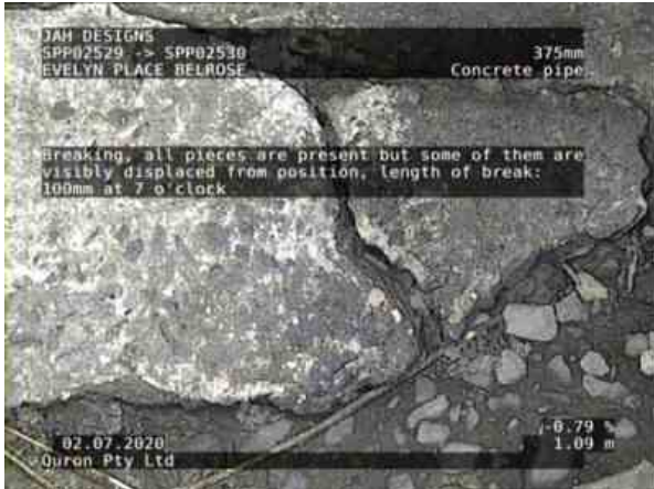
SPI01992_8b654be4-ce45-454c-993e-9086569f6f1d_20200702_122251_886.jpg, 00:01:03, 1.09 Breaking, all pieces are present but some of them are visibly displaced from position, length of break: 100mm at 7 o'clock
