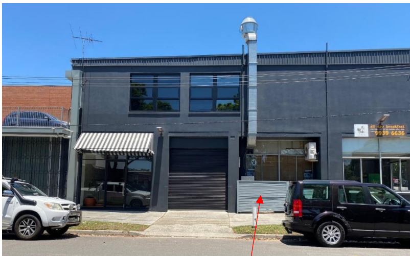
Communal Bin Storage Area for Lots 1 and 2
