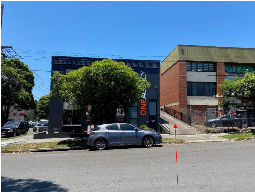
Photograph of the site from Ada Avenue – note vehicular ramp to parking
