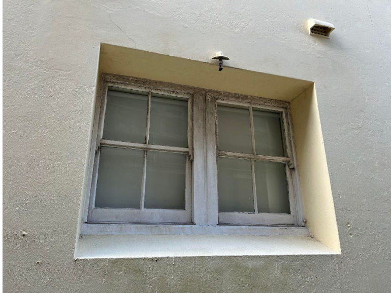
Figure 4 – Example of an original Window – Source: Hector Abrahams Architects
