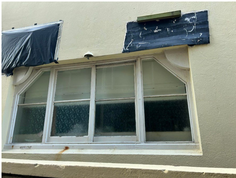
Figure 5 – Example of a replaced Window (non-original frames) – Source: Hector Abrahams Architects
