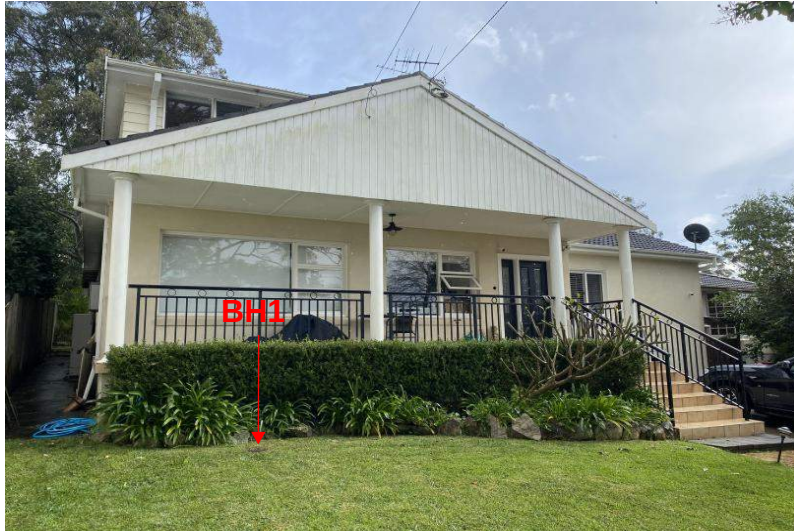
Position of BH1 in front garden area
