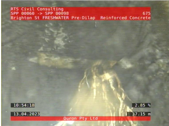
1, 00:14:50, 37.15 Fine roots--a relatively small number of flexible minor roots, at joint, Obstruction: <5% at 6 o'clock
