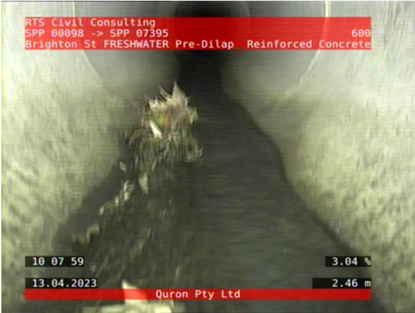
1, 00:00:59, 2.46 Tap roots--a small number of major roots (10mm or greater) without a significant mass of fine root, at joint, Obstruction: 5-20% from 6 o'clock to 8 o'clock, Start #
