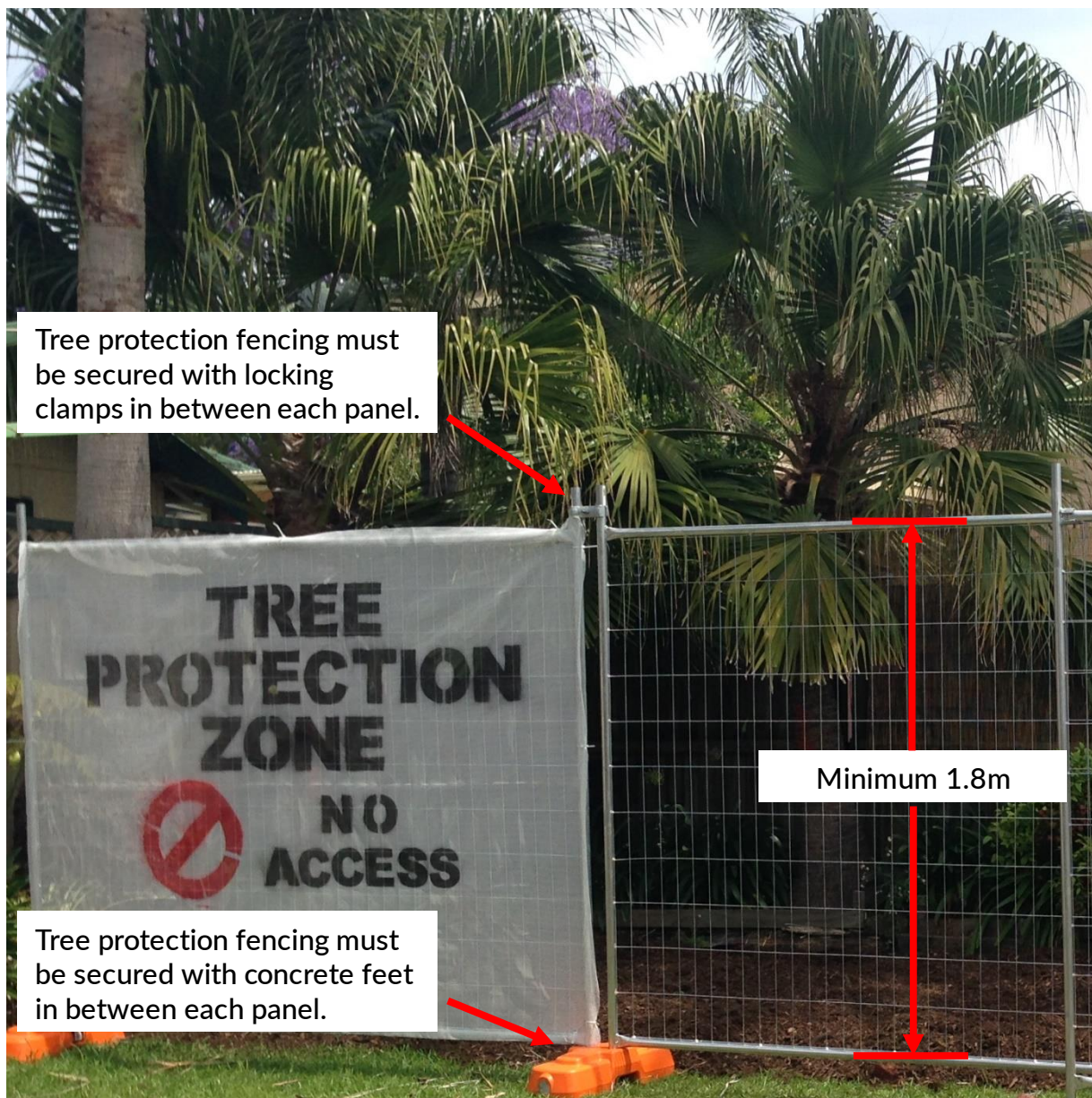
An Example of Temporary Fencing
