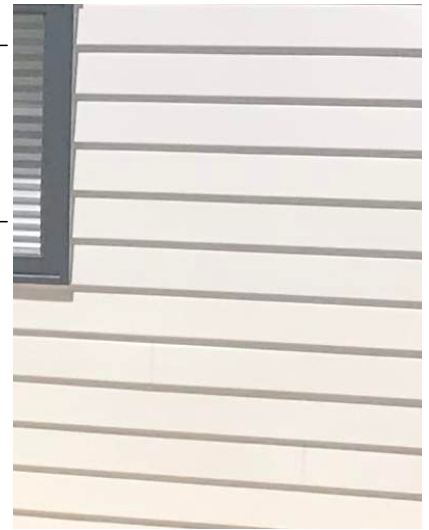
1 - Weatherboard to match existing
