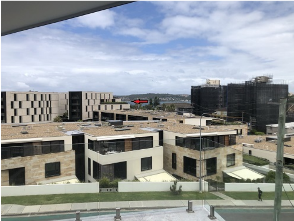
Image 2 - View from first floor balcony
