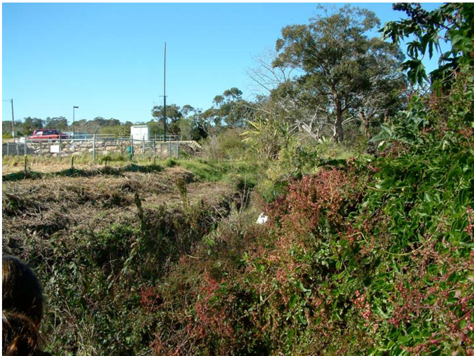
Plate 4: Narrabeen Creek showing the condition extent of the overgrown vegetation.
