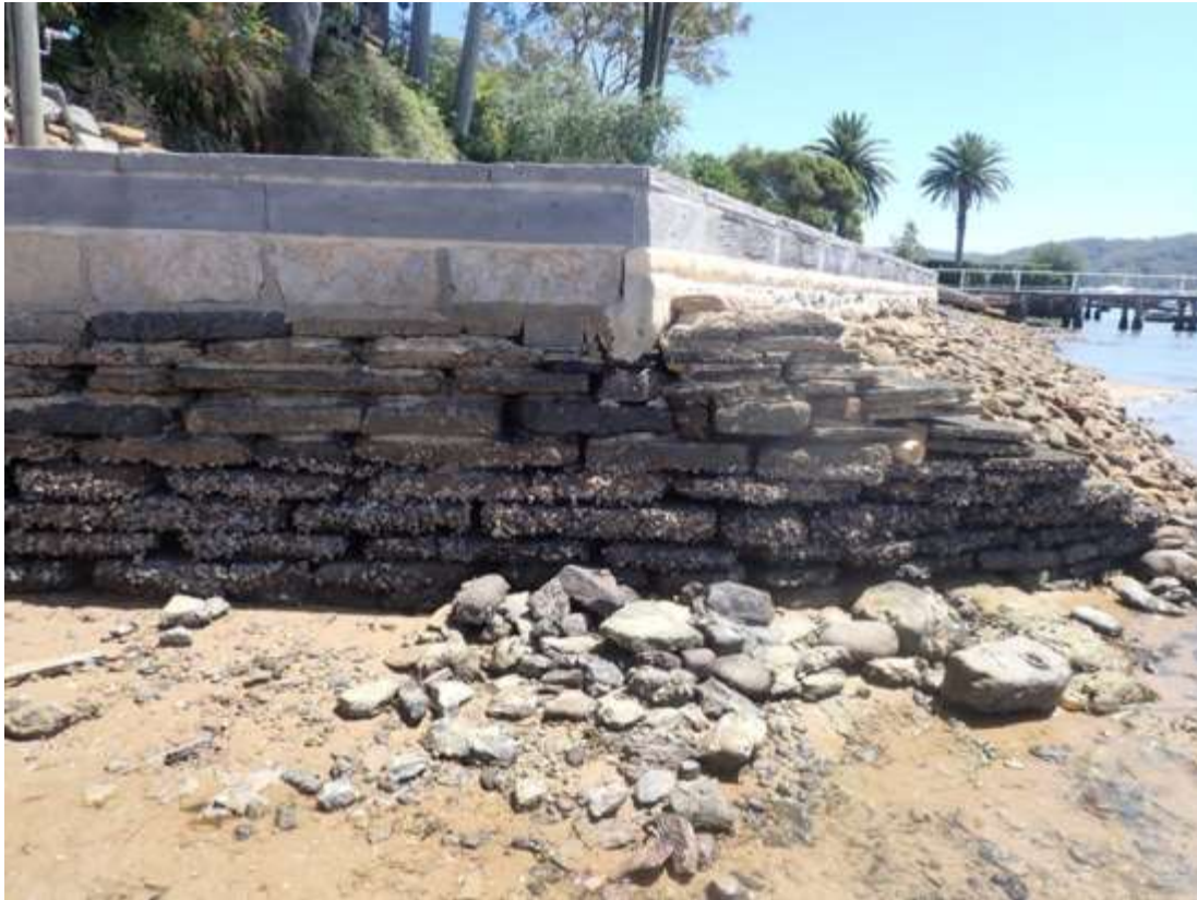
Figure 6 View of common boundary between the two properties showing block sandstone seawall along the north-east edge of No 1744 property to be replaced and placed river cobbles lining the front edge of the seawall (to be retained).
