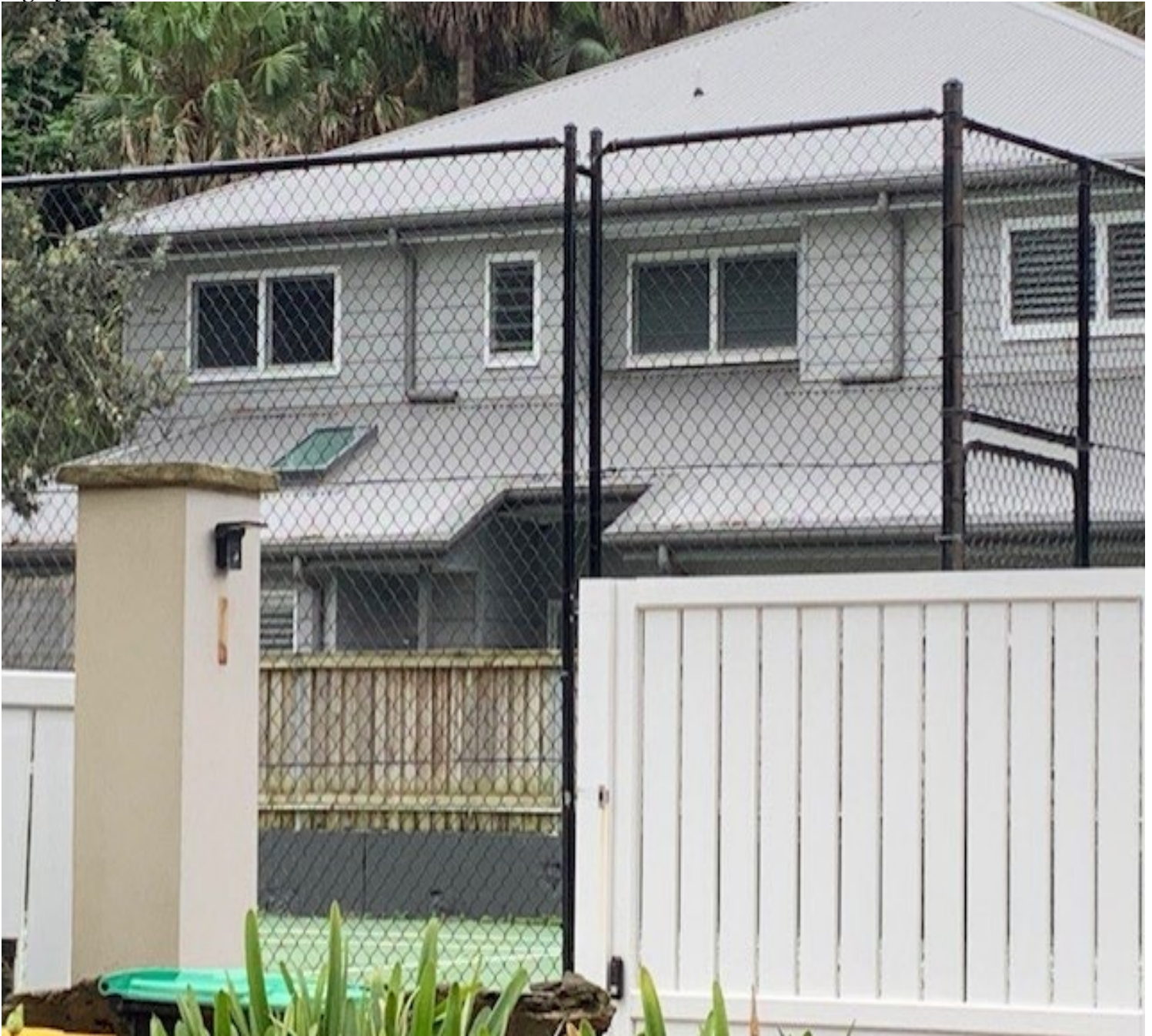
Figure 6 – Photo taken from Allen Avenue showing the tennis court and associated tennis court fencing in photo 5. Given the colour of the dwelling house at no. 4B Allen Avenue, the black 3 metre high fence is highly visible
