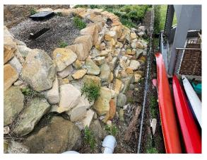
It is understood from the supplied survey drawing that the walls were complete prior to 6<sup>th</sup> September 2019 with several photos of the location during construction supplied by the site owners indicating that the foundation below the main portion of the walls is sandstone bedrock.
