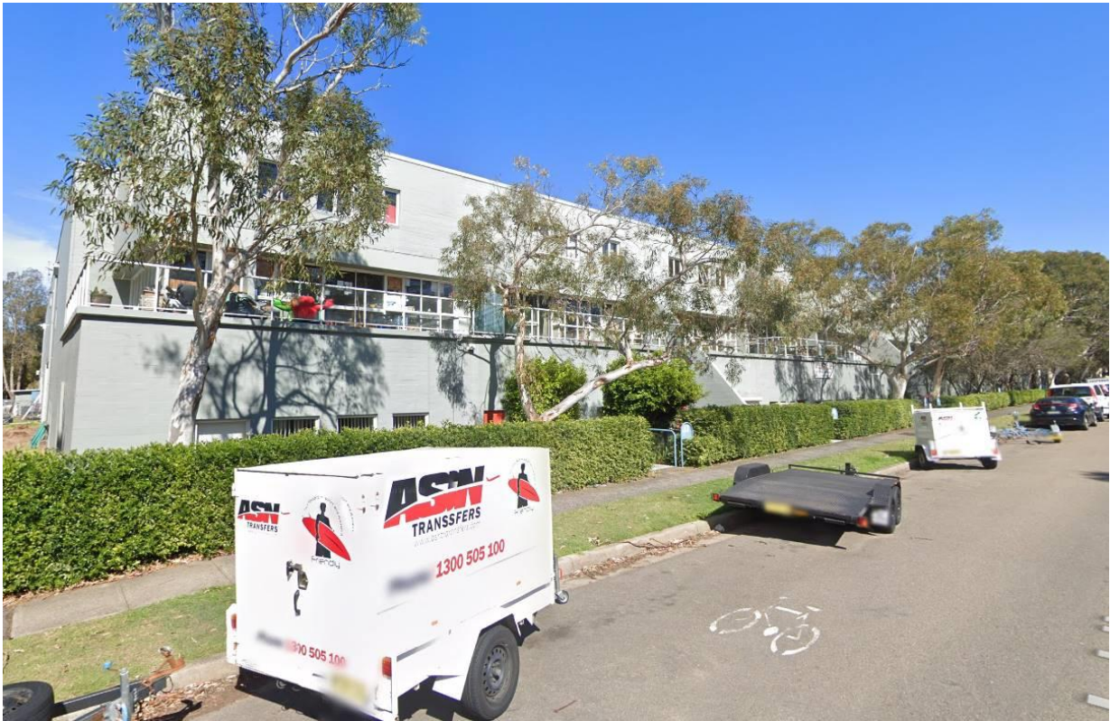
Figure 5 – View of the property to the west of the subject site No. 6 Ponderosa Parade
