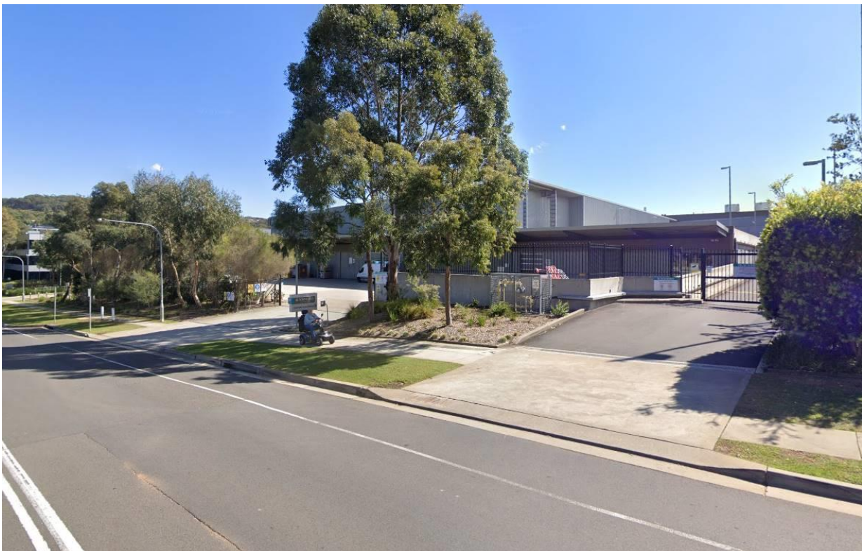
Figure 6 – View towards the Blackmores campus directly opposite the subject site
