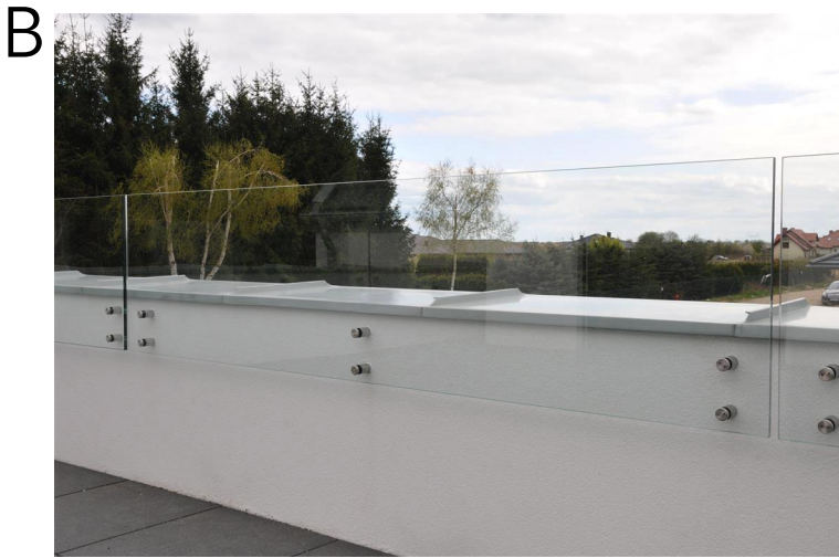
NEW GLASS PANEL BALUSTRADE TO OWNER'S REQUIREMENTS
