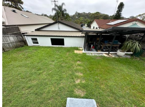
Photo 2: Rear of the dwelling facing north-east.
