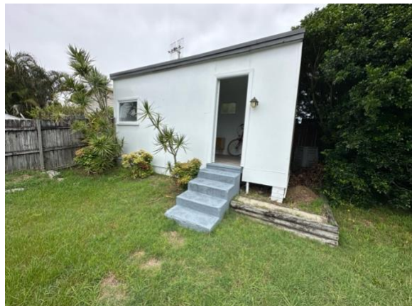
Photo 3: Existing studio at the rear of the site.
