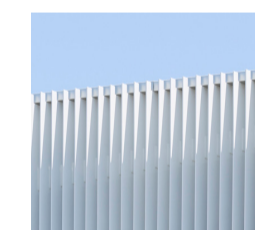
LO-2 External Louvres - Fixed Powdercoat White
