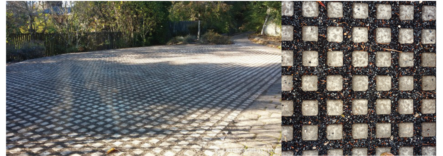
Permeable paving grasscrete for carpark
