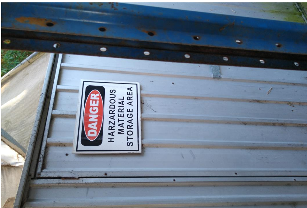
Photo 14 – Hazardous Materials Storage Cupboard
