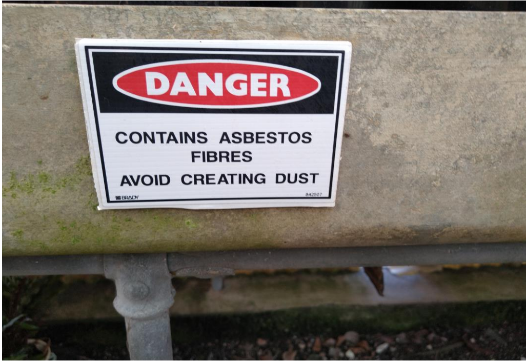
Photo 5 – Asbestos danger sign inside plant nursery
