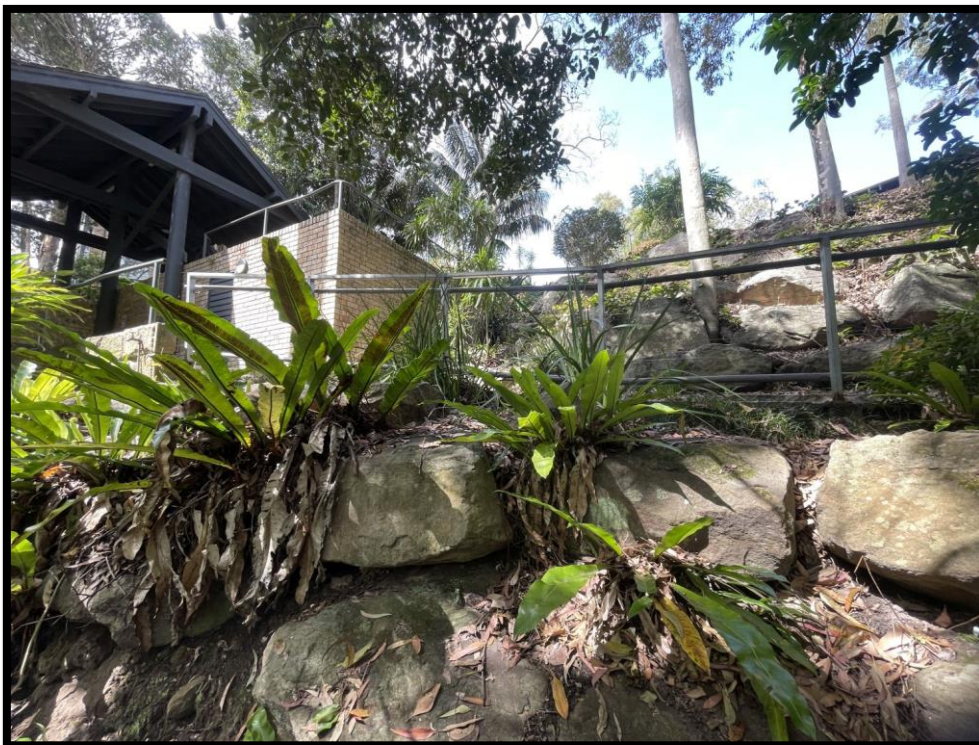
Plate 3 – Lower boulder wall, looking north-east
